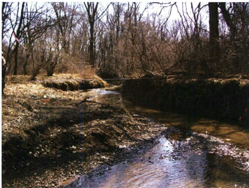
Figure 5-14. View of AR3-XS2 (facing downstream).
