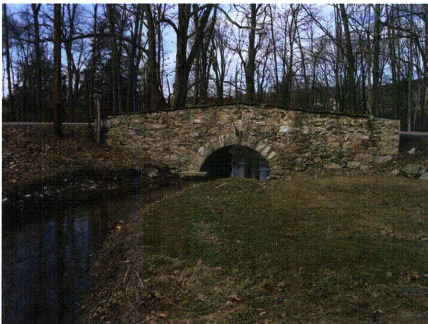
Figure 4-1. View of the south Market Street bridge crossing (facing downstream).
