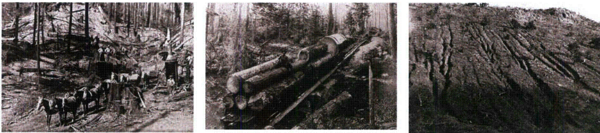
Figure 3-2. Indiscriminate land clearing caused massive erosion from hillsides.
