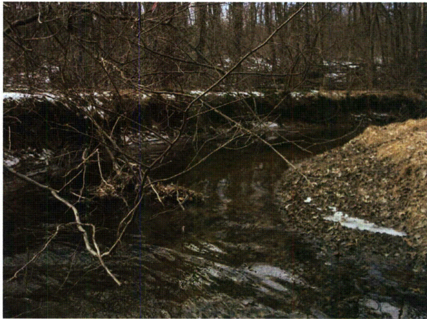
Figure 4-11. View of typical stream conditions showing bank erosion between Market Street and Beach Grove Road.
