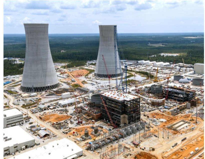
Vogtle construction site
