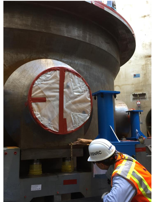
Inspector in the field with Unit 3 reactor vessel
