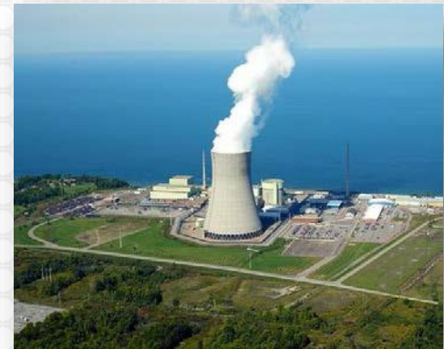
Nine Mile Point ~ Courtesy Constellation Energy
