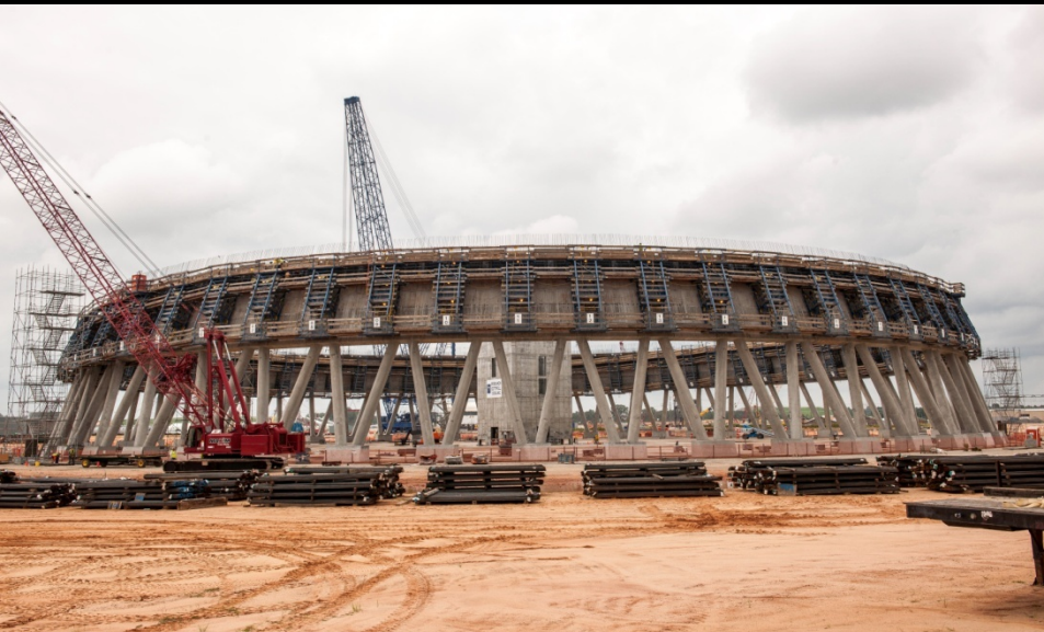
Plant Vogtle Unit 3 cooling tower construction
