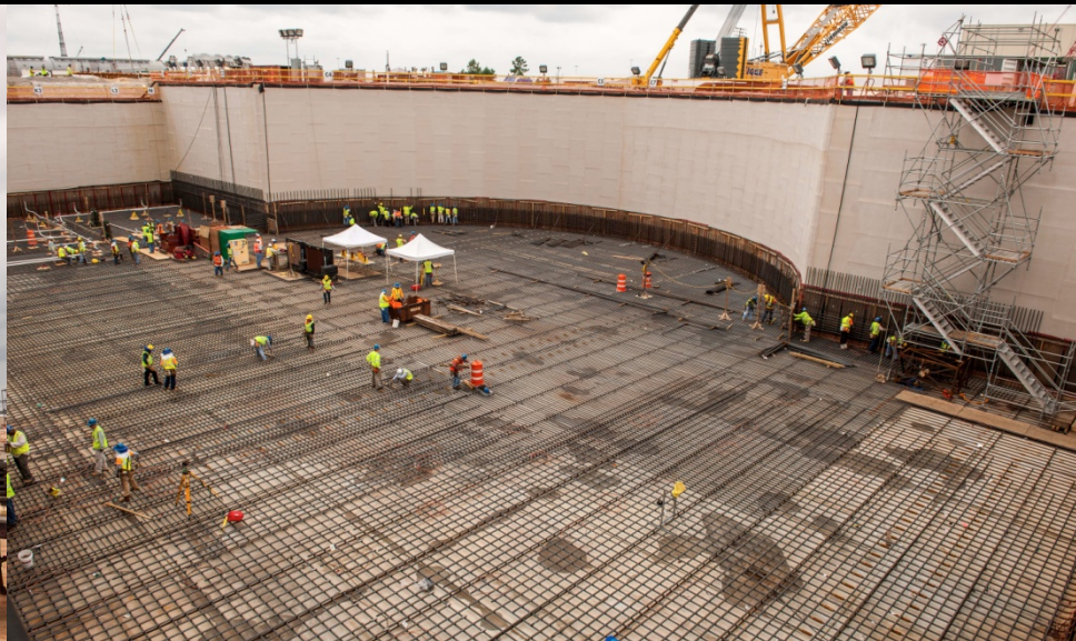
Plant Vogtle Unit 4 nuclear island rebar placement
