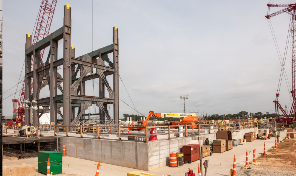
Plant Vogtle Unit 3 turbine building construction
