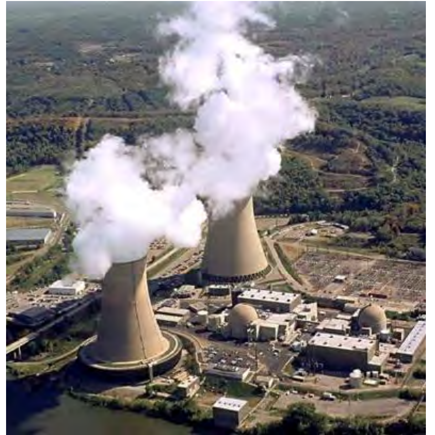
Beaver Valley Power Station (Units 1 and 2) in Shippingport, PA Photo: First Energy
