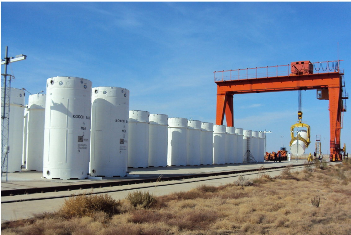
Massive containers hold spent nuclear fuel at safe and secure dry storage facilities. This photo shows, at right, a dry cask recently loaded with spent fuel being lifted from a horizontal transporter to be placed vertically on a specially designed storage pad. Photo courtesy of Sandia National Laboratories.
