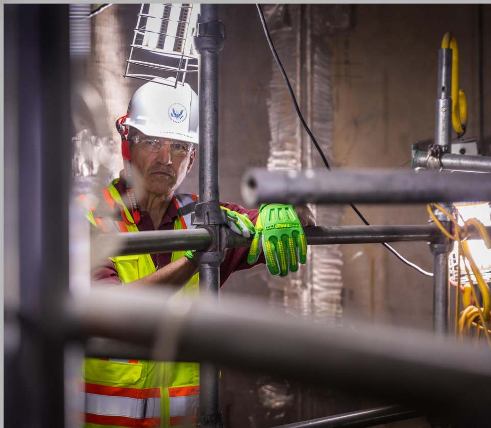
NRC Division Director Chris Miller observes new construction activities at Vogtle Units 3 and 4 in Georgia.
