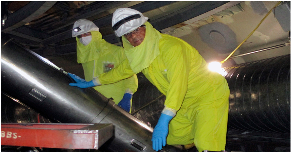
NRC Region IV Administrator Scott Morris (right) and Senior Resident Inspector Andrew Siwy (left), dressed in protective gear, examine the plant's drywell during a refueling outage at the Cooper nuclear power plant in Brownville, Nebraska. Photo courtesy of Nebraska Public Power District.
