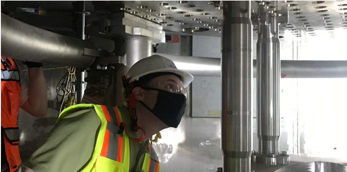
NRC Commissioner Jeff Baran observes the reactor vessel head inside Unit 4 containment, currently under construction at the Vogtle site in Georgia.
