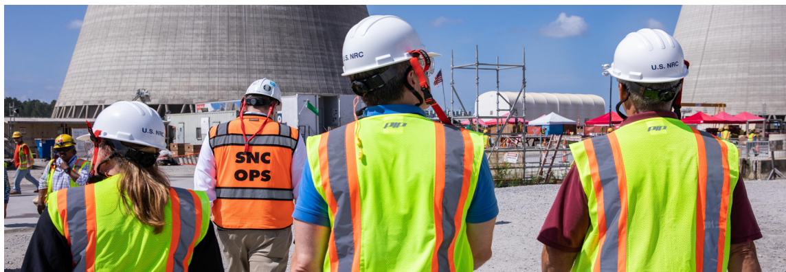
NRC senior leaders observe new construction activities to ensure NRC regulations are being met at Vogtle Units 3 and 4 in Georgia.
