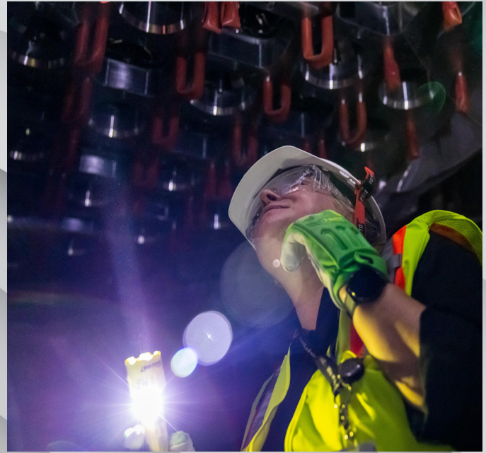
NRC Office of Nuclear Security and Incident Response Director Mirela Gavrilas observes new construction activities at Vogtle Units 3 and 4 in Georgia.
