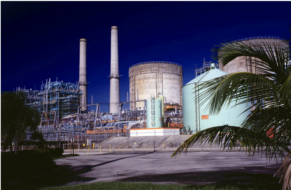
Turkey Point nuclear power plant in Florida was the first U.S. plant to be approved by the NRC for subsequent license renewal, or an additional 20 years of operation, for a total lifespan of 80 years.
