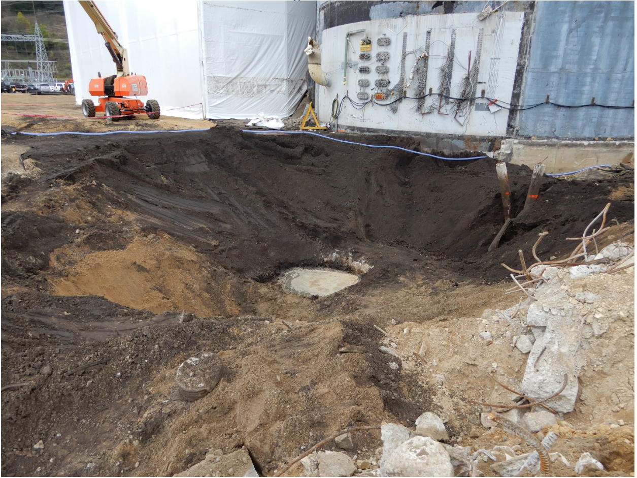
L1-SUB-CDR following Backfill September 2017
