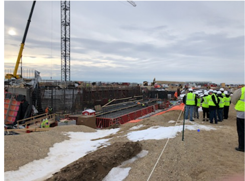
SHINE Construction Site in February 2020
