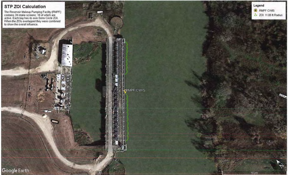
FIGURE 9: Expected Zone of Influence at the RMPF Cooling Water Intake Structure
