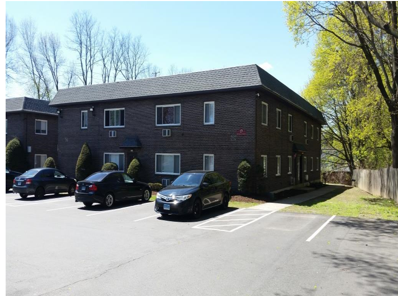
Figure A-6. Northeast Corner of 320 Queen Street
