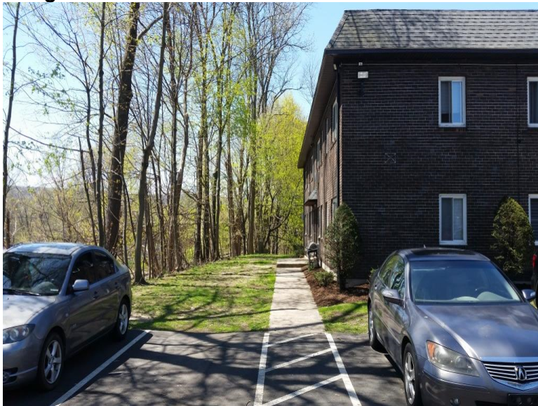
Figure A-7. Southeast Corner of 332 Queen Street
