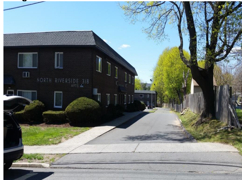
Figure A-4. Northeast Corner of 318 Queen Street
