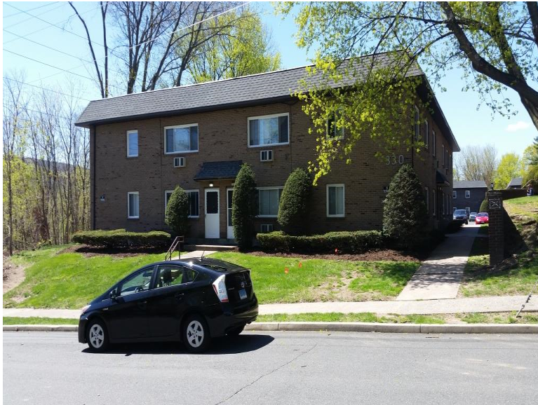
Figure A-1. Eastside of 330 Queen Street
