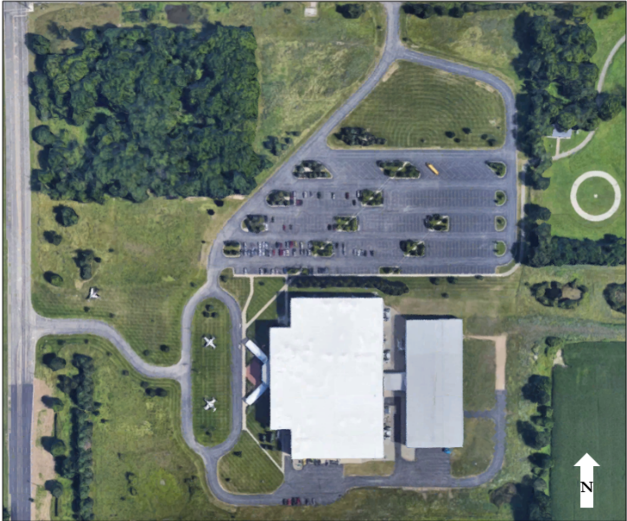
Figure 3. Aerial View of Air Zoo Main Campus (Google Earth Pro 2017)
