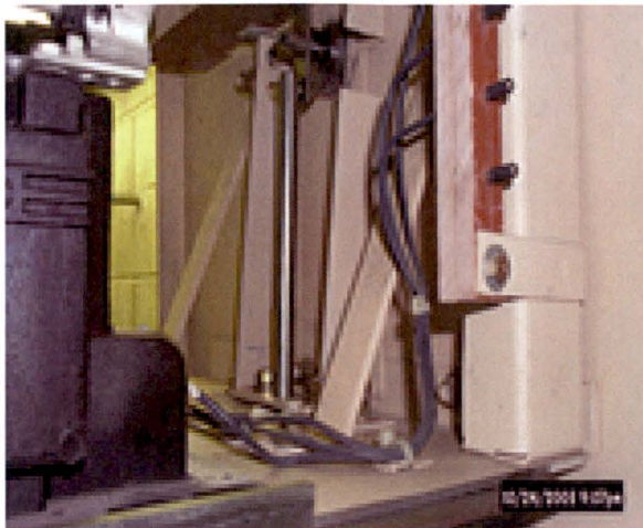
Figure 10 – Potential Transformer (PT) Cubicle Internals Examples
