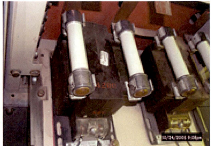
Figure 10 – Potential Transformer (PT) Cubicle Internals Examples
