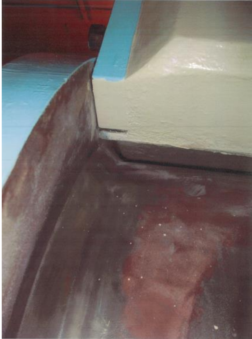
Figure 1.16-3 Weld 1-CP-206-CSP-W2 Limitations
