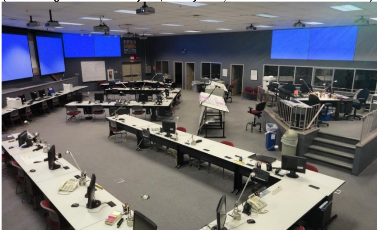
Coatesville EOF Main Operations Room (in the background are the Maryland, Pennsylvania, and Protective Measures Rooms)
