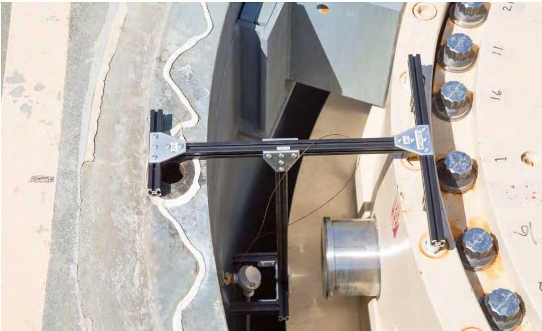
2. Liner exam fixture supporting plumb bobs (shown around temperature probe in this location)
