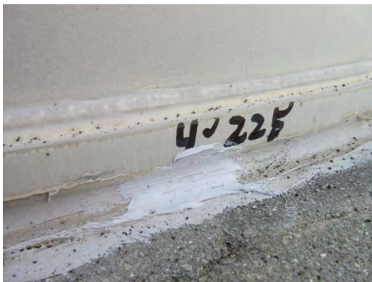
17. Cell 4 Caulking As-Left
