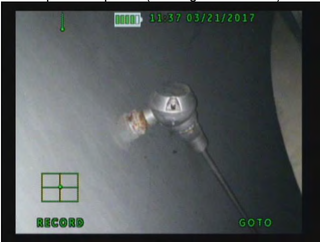
3. Temperature probe (no longer in-service)
