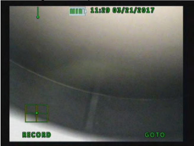
14. Looking down overpack at seismic shim
