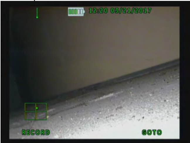
11. Overpack and Vault Liner Bottom with Debris
