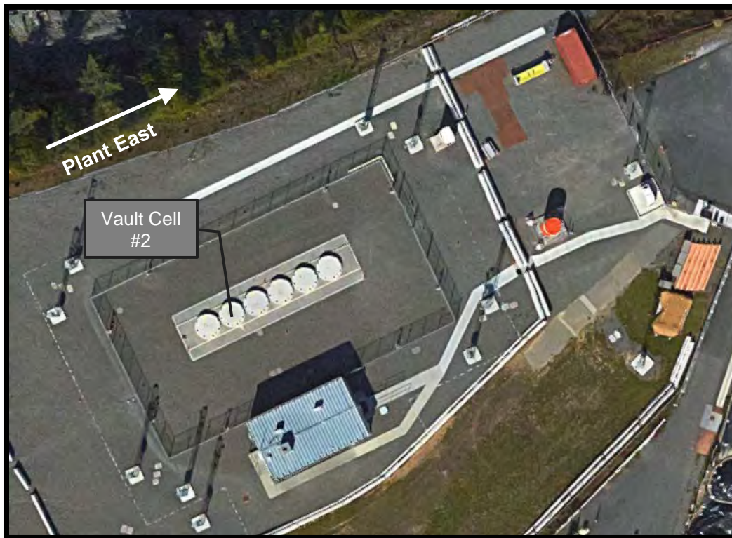
Figure 3: HB ISFSI Aerial View with Vault Cell #2 Identified
