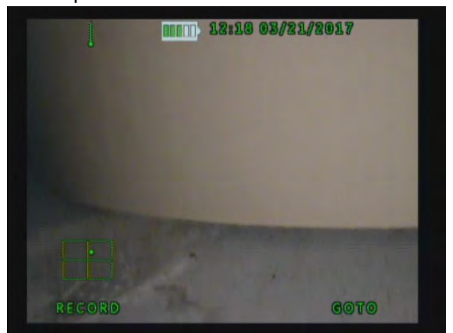
6. Overpack and Vault Liner Bottom
