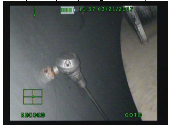
4. Temperature probe (no longer in-service)
