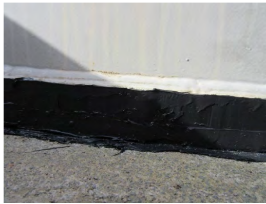
16. Cell 2 Caulking As-Left
