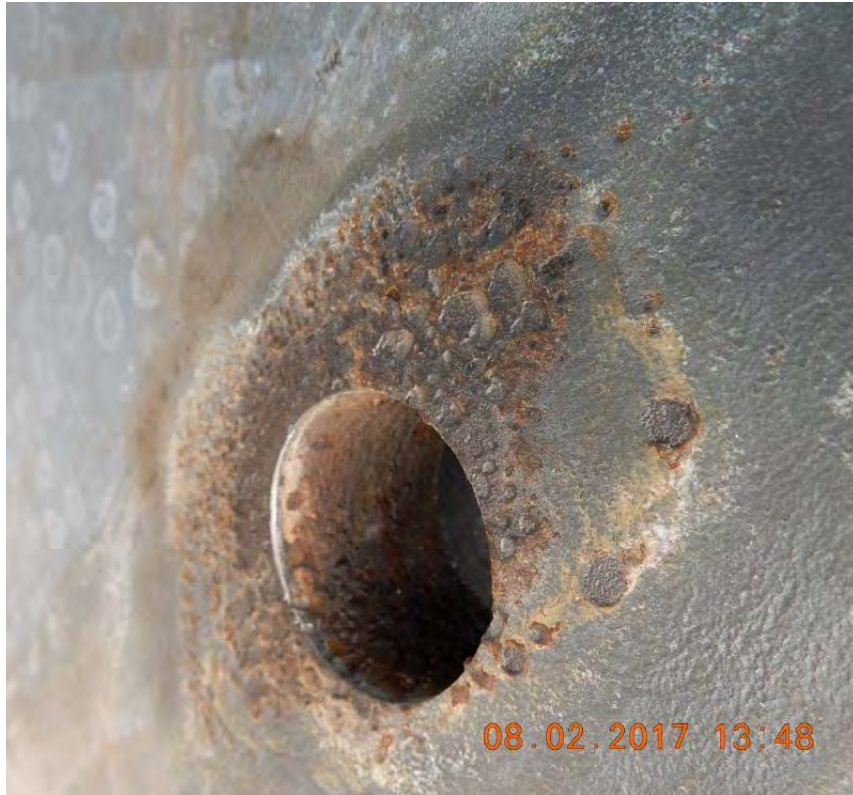
9. Hole #5 after cleaning
