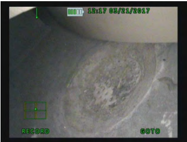
5. Vault Liner Bottom and Vault Drain
