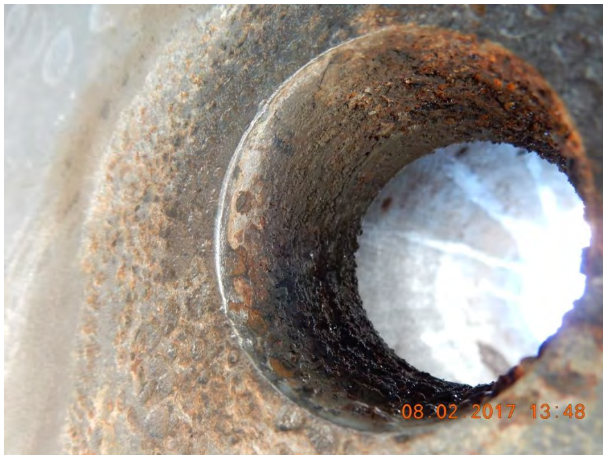
10. Hole #5 after cleaning
