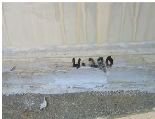
18. Cell 4 Caulking As-Left
