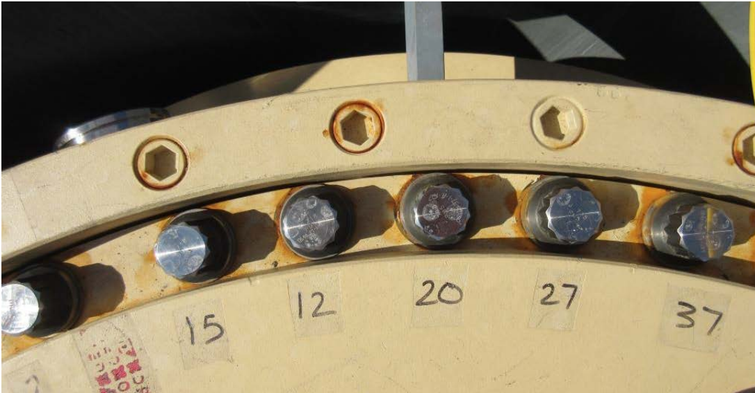
16. Rust staining around overpack lid closure bolting and around top flange plug set screws
