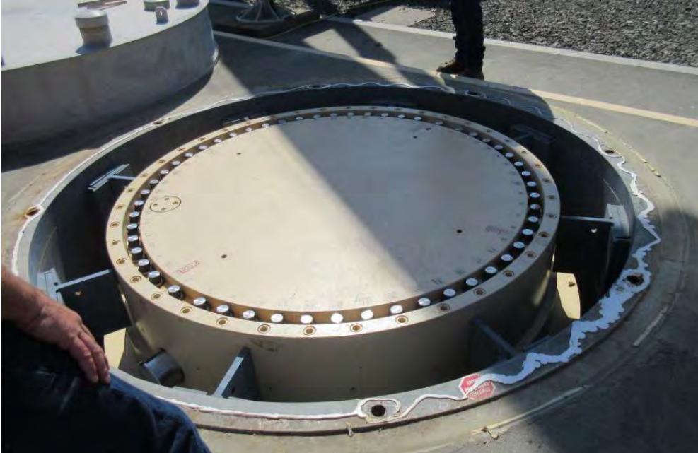
14. Upper portion of overpack exposed for direct visual examination
