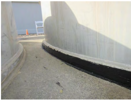
15. Cell 2 Caulking As-Left
