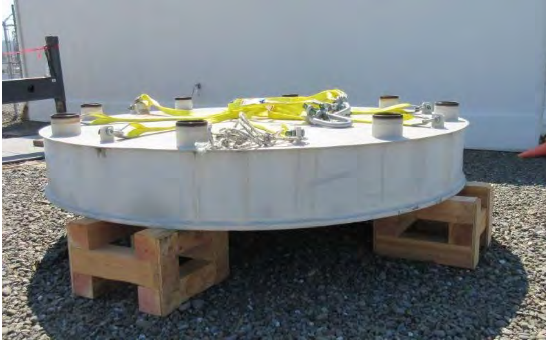
5. Removed lid on cribbing
