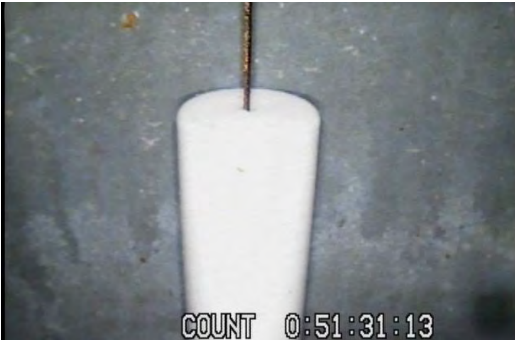
53. Scan 2 rust spot (for size comparison, the wire cable supporting the plumb bob is 1/32" dia.)
