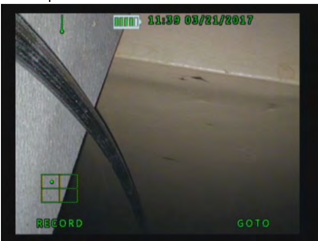
5. Overpack and seismic shim
