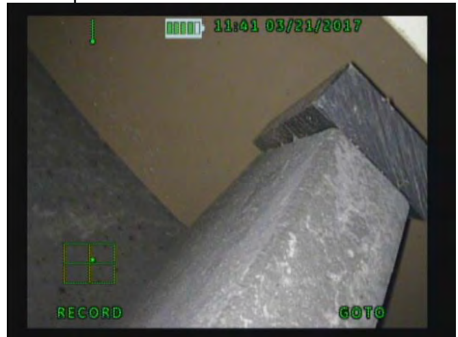
6. Overpack and seismic shim
