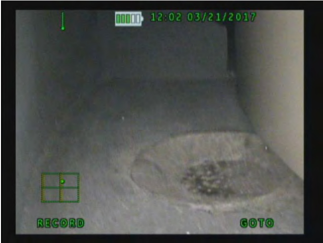
7. Vault Liner Bottom and Vault Drain
