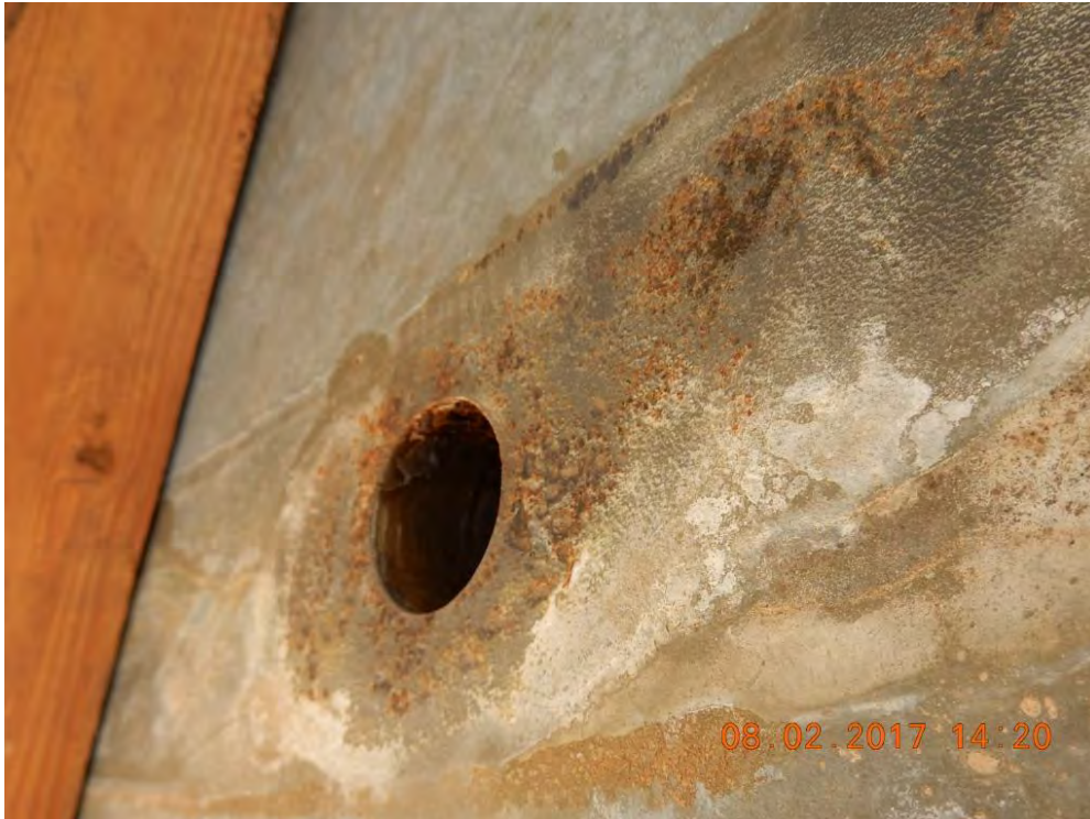
11. Hole #3 after cleaning
