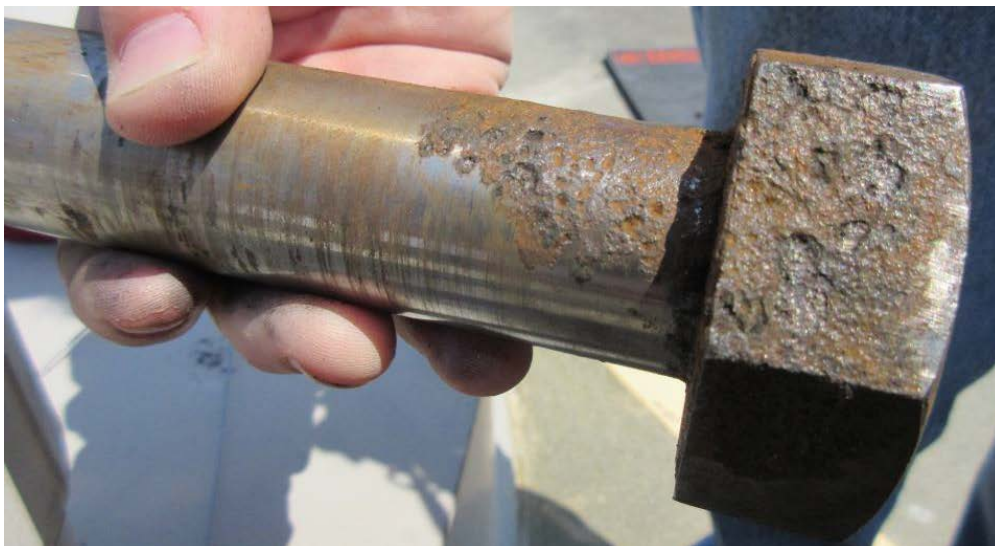
66. Removed bolt following cleaning (pitted bolts replaced)
