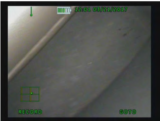
5. Vault Liner Bottom
