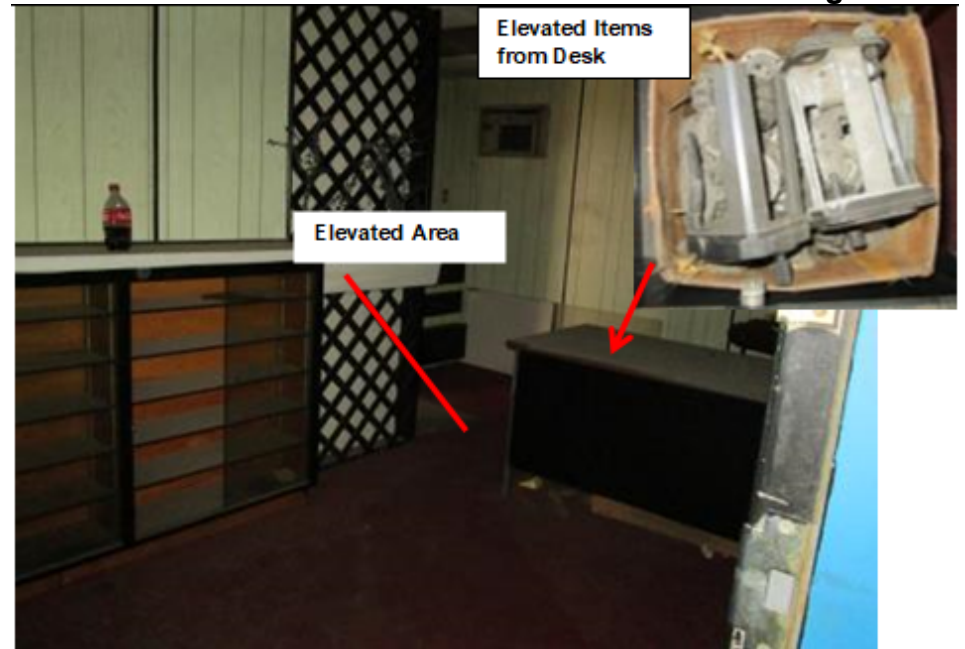
A-16. Hangar 13 Upper Level Offices
