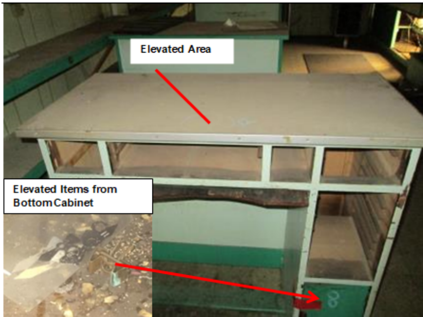
A-17. Hangar 13 Upper Level Offices
