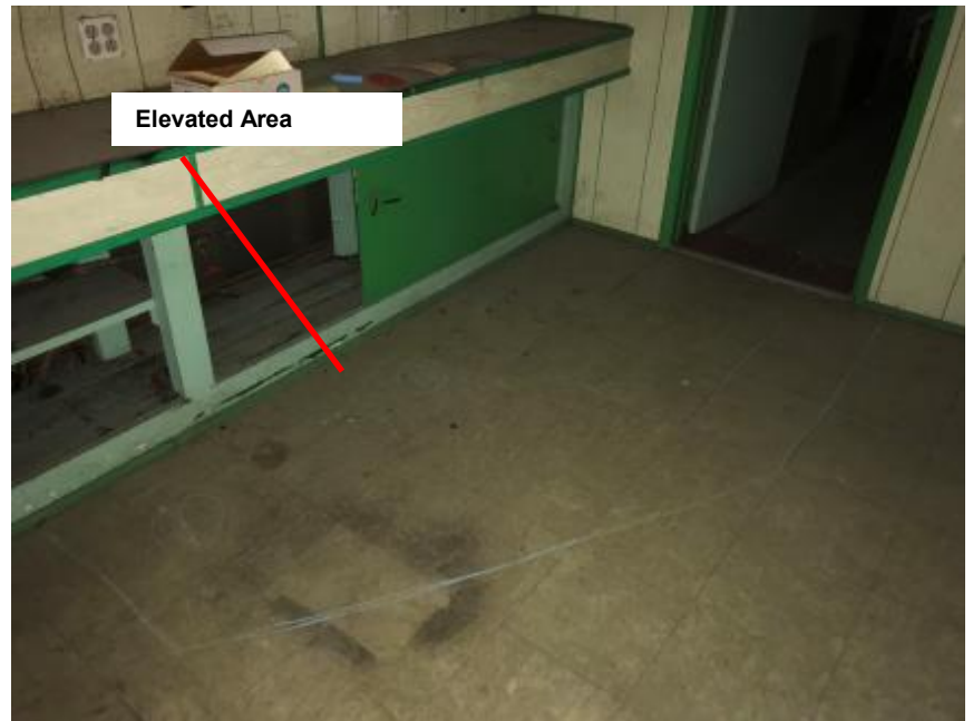
A-18. Hangar 13 Upper Level Offices
