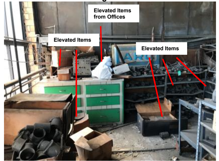
A-12. Elevated Items Placed on Roof of Offices within Hangar 13
