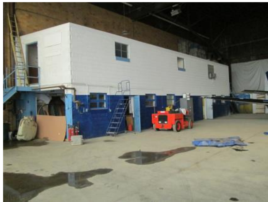
A-2. Hangar 9 Offices
