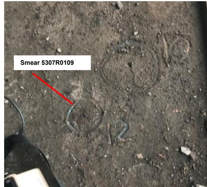
A-14. Elevated Areas on Roof of Offices within Hangar 13
