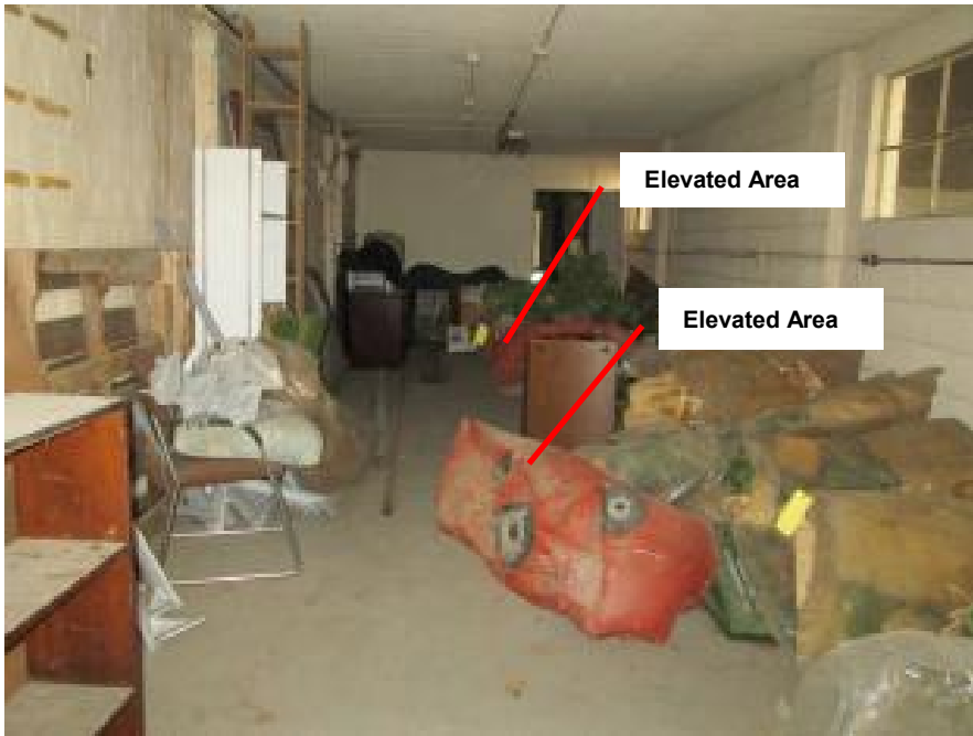
A-5. Hangar 9 Upper Level Offices
