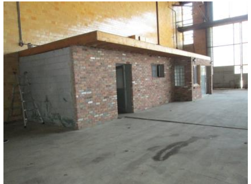
A-8. Hangar 10 Lower Level Offices/Roof
