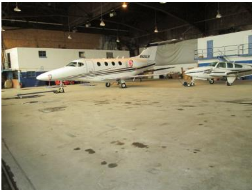
A-1. Hangar 9 Bay Looking Southeast
