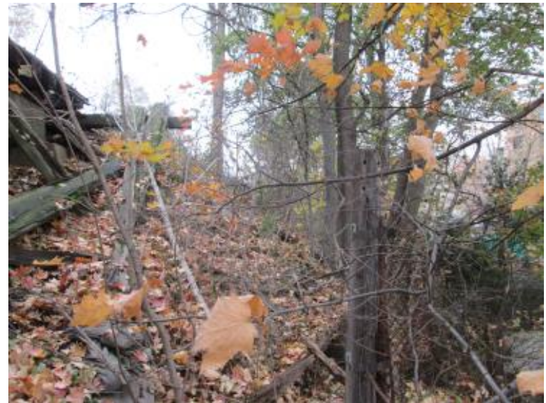
Figure A-10. Eastern Embankment Under Abandoned Railroad
