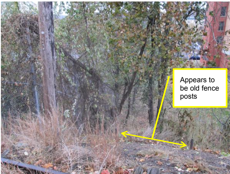
Figure A-11. Eastern Embankment South End
