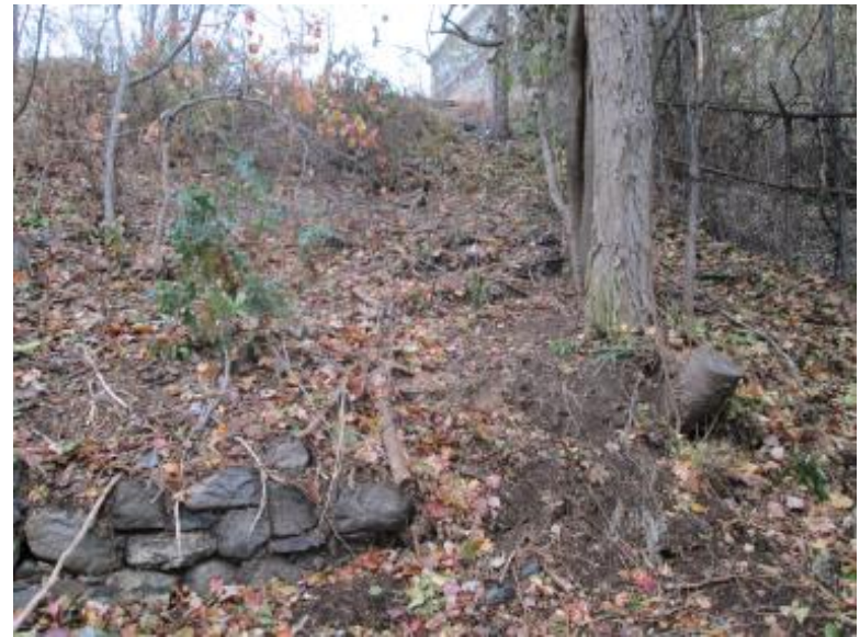
Figure. A-6. Eastern Embankment South End Looking Up (East)
