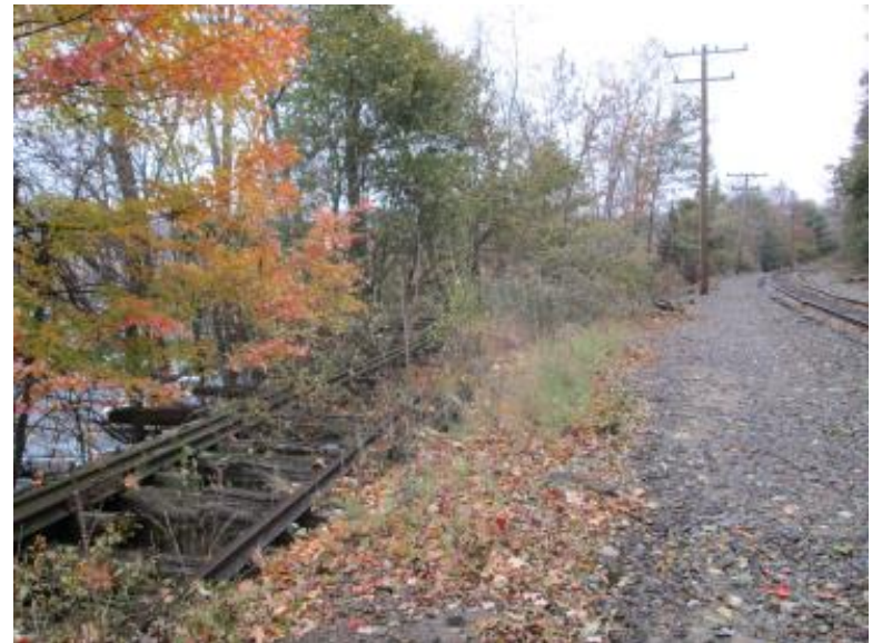
Figure A-4. Abandoned Railroad (left) in Eastern Embankment
