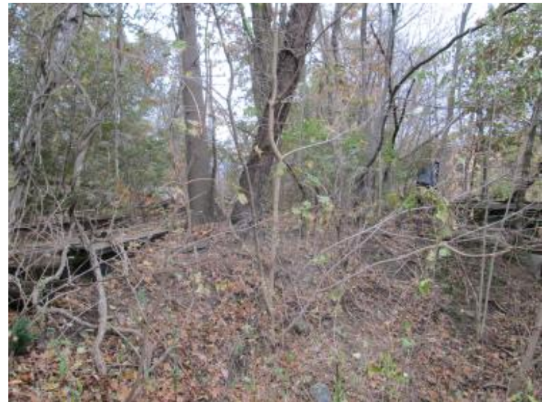
Figure A-2. Eastern Embankment East Side North End
