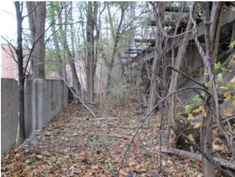
Figure A-9. Eastern Embankment Under Abandoned Railroad
