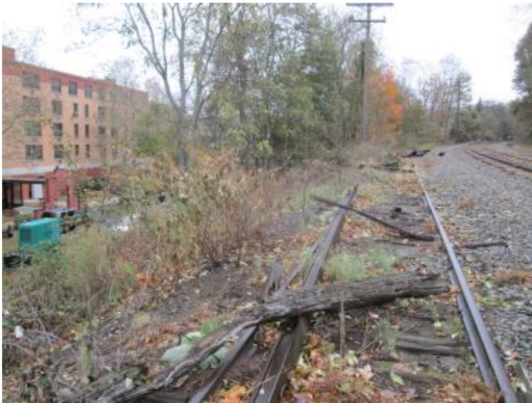
Figure A-5. Eastern Embankment East Side South End
