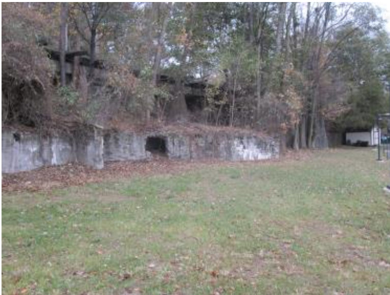
Figure A-1. Eastern Embankment West Side North End
