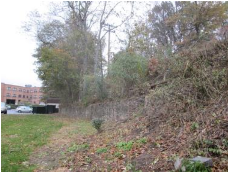
Figure A-7. Eastern Embankment West Side South End
