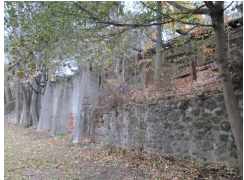
Figure A-8. Eastern Embankment West Side Midway
