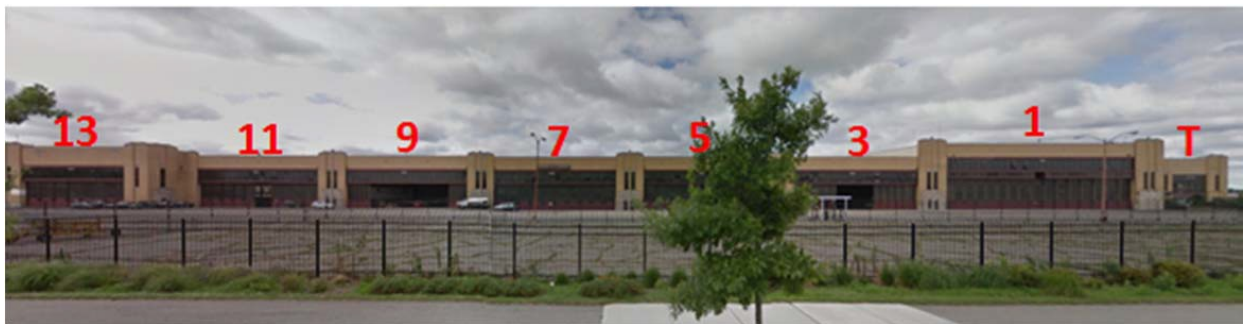
Figure 3. Executive Terminal, view from Connor Street, showing location of original terminal/administration area (T) and approximate locations of odd-numbered hangars (Google Earth, 2017).
