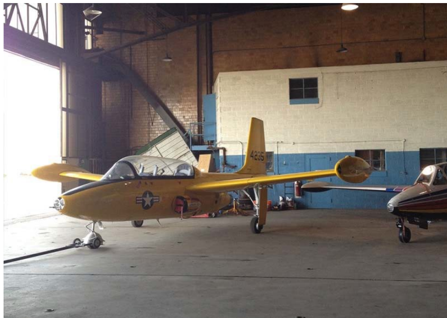
Figure 5. Example of “rooms” inside hangars of the Executive Terminal at Detroit City Airport. Note the blue and white two-story block structure in the hangar bay.
