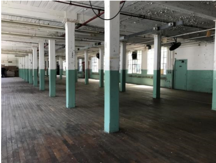
A-7. Former Lux Clock Company Third Floor
