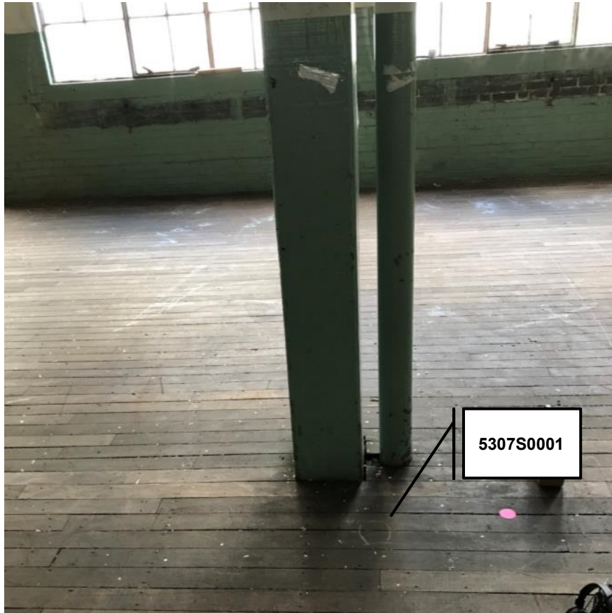
A-5. Former Lux Clock Company Third Floor Elevated Area
