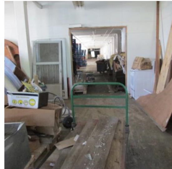
A-10. Former, Lux Clock Company Second Floor
