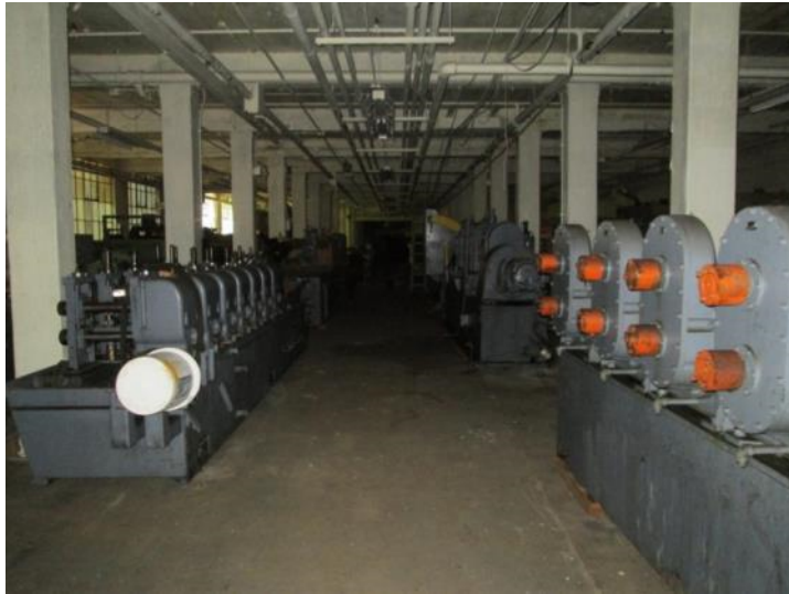
A-11. Former Lux Clock Company First Floor (Basement)
