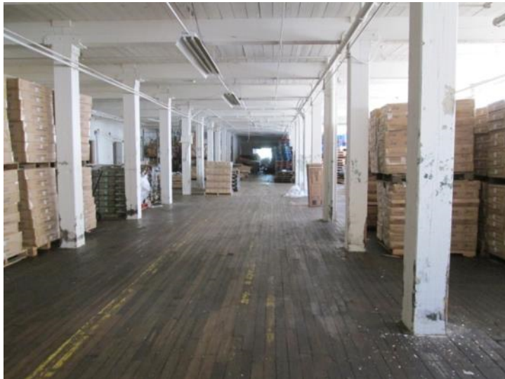
A-9. Former Lux Clock Company Second Floor
