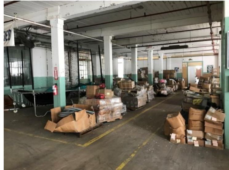
A-8. Former Lux Clock Company Third Floor
