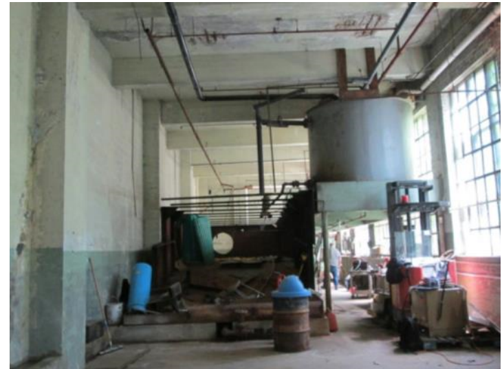
A-14. Former Lux Clock Company Sub-Basement
