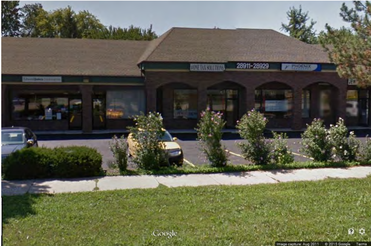
Figure 2. Former location of Aerospace Innovations, 28919 Seven Mile Road in Livonia, MI (now One Tax Solutions) (Google Earth, 2015)
