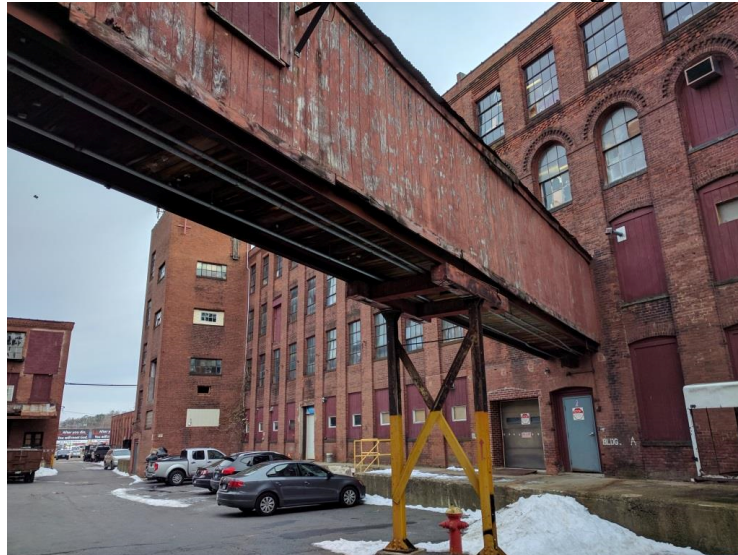
A-9. Bridge Between Building A and W
