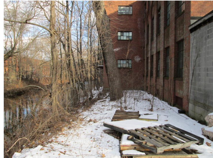
A-10. Access Limitations North of Building X and W
