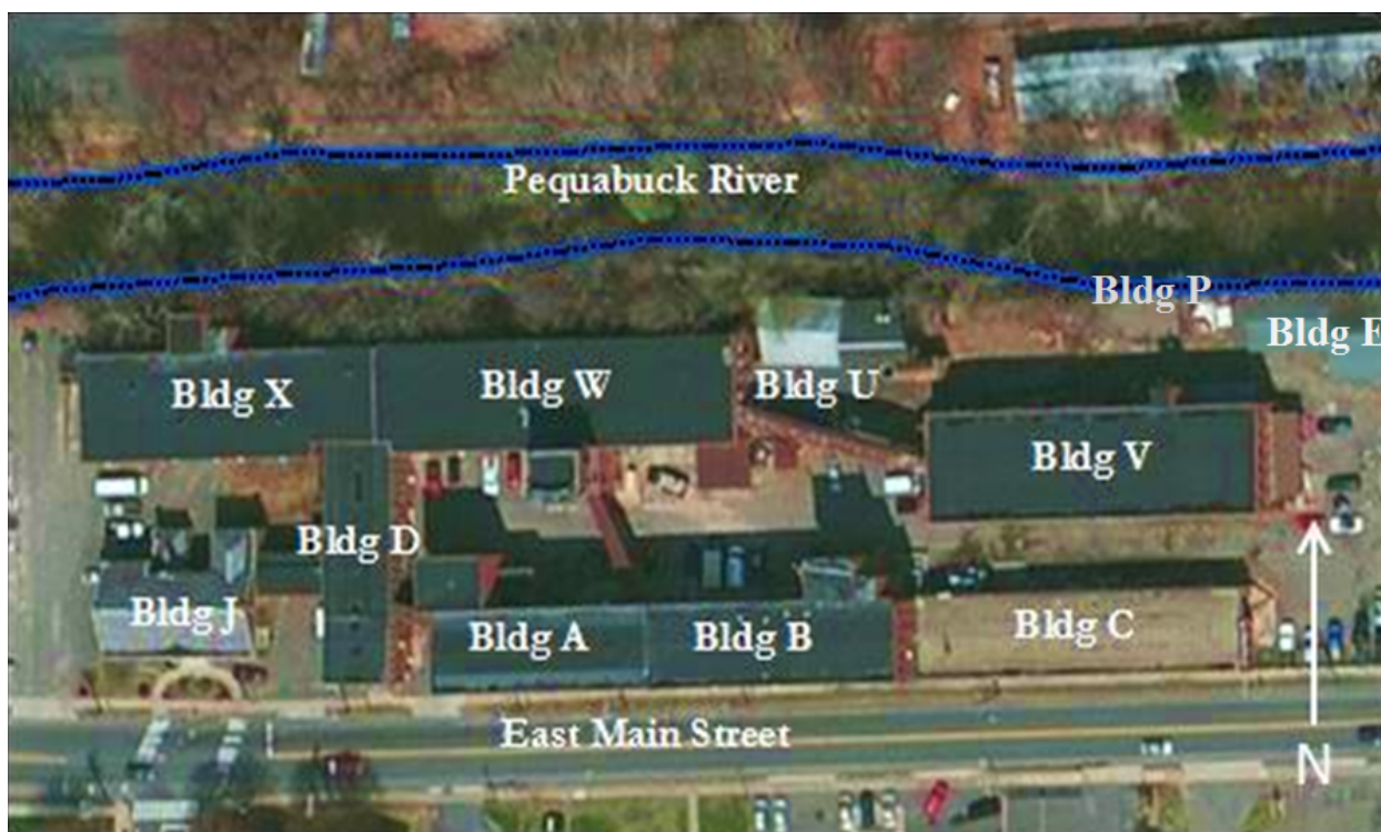
Figure 1. Aerial Photo of the Sessions Clock Company at 61 East Main Street
