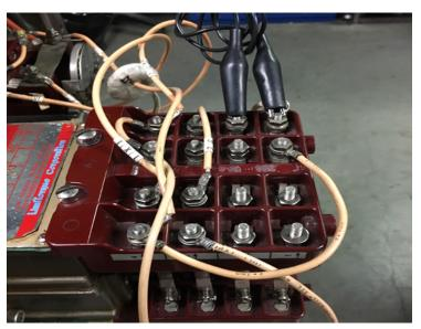
Typical MOV Limit Switch finger base with Jumper
