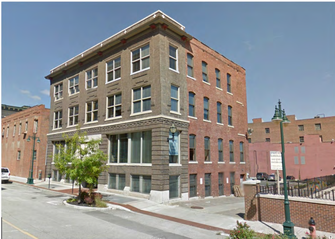
Figure 6. Side of Adler Building with sign for IAAO World Headquarters (Google Earth, 2014)
