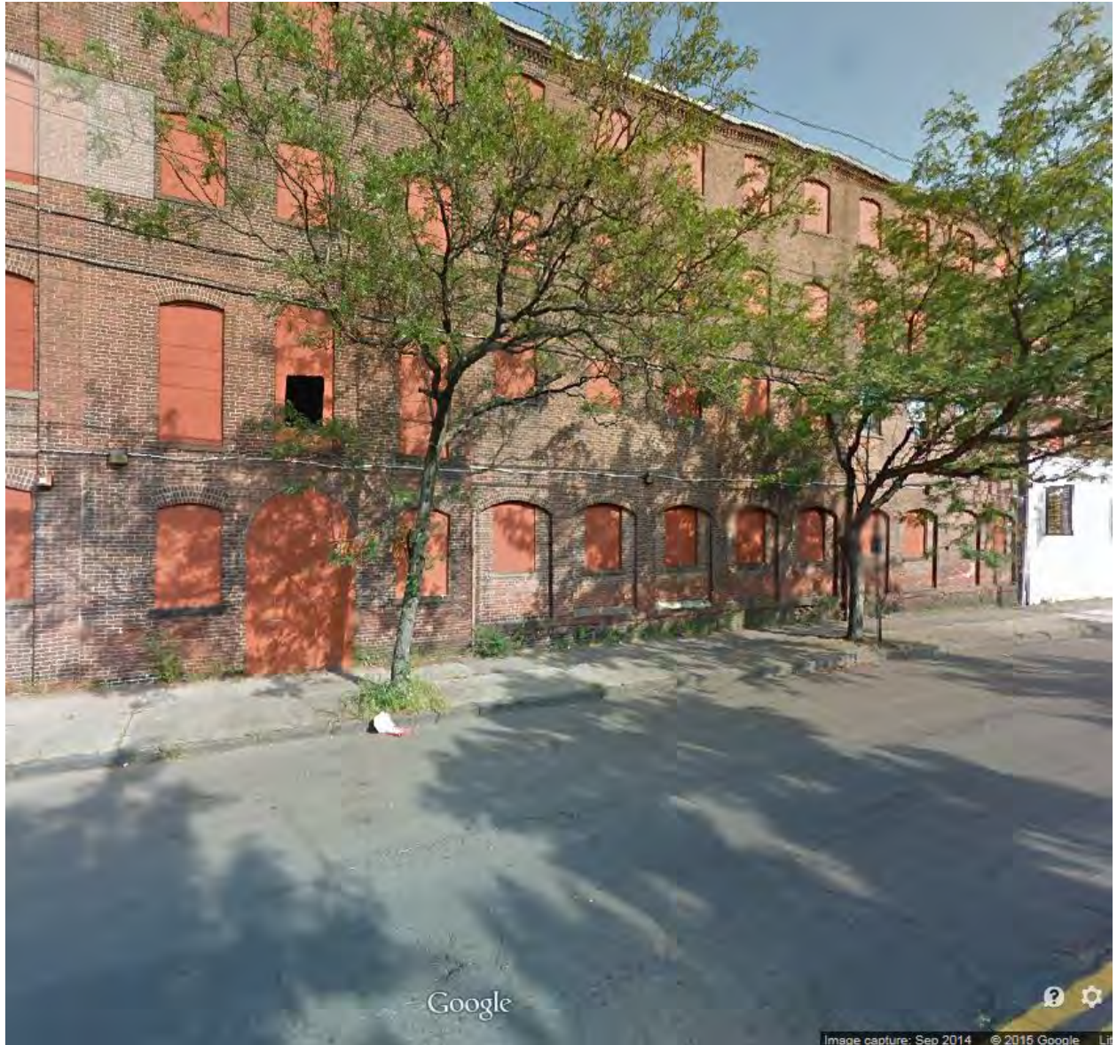
Figure 3. Former New Haven Clock Company Building (Google Earth, 2014)
