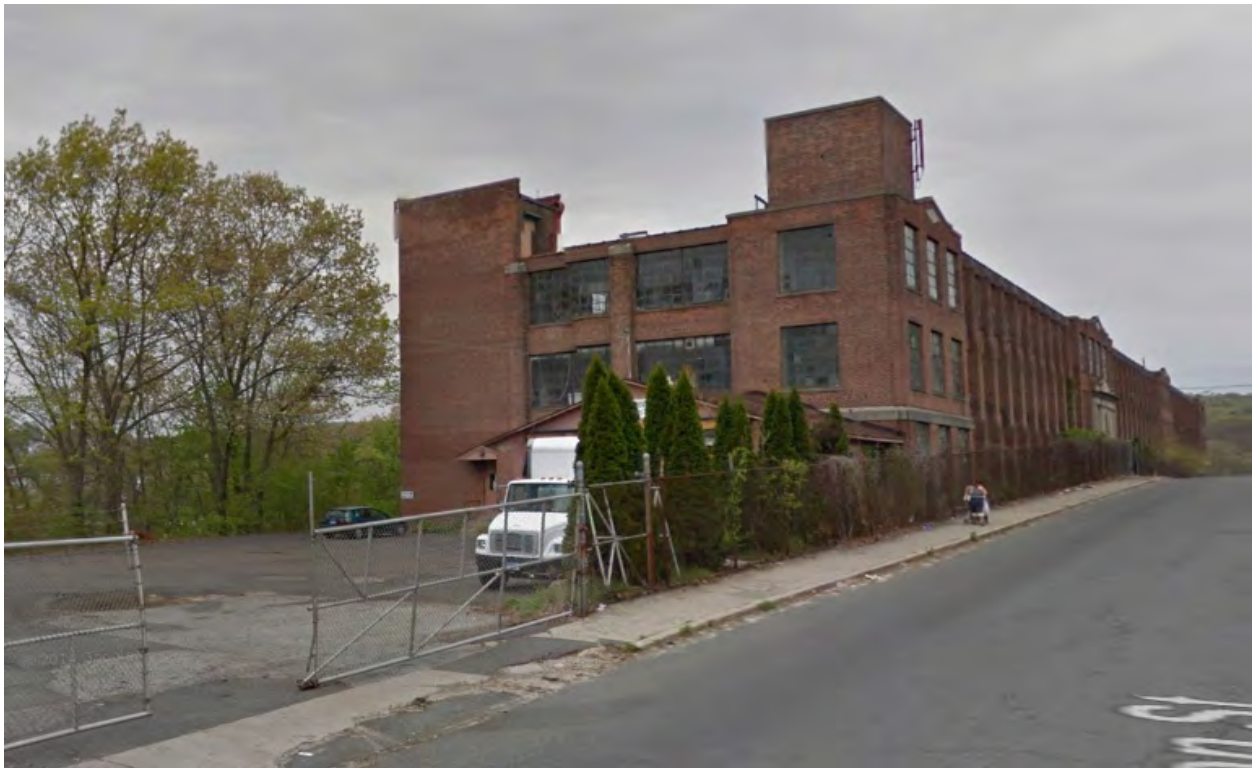
Figure 4. Shipping entrance to former Lux Clock Company (Google Earth, 2015)
