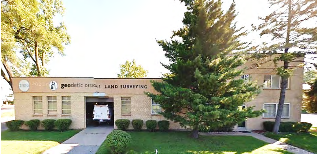
Figure 2. 2300 North Grand River Avenue (Google Earth, 2015)
