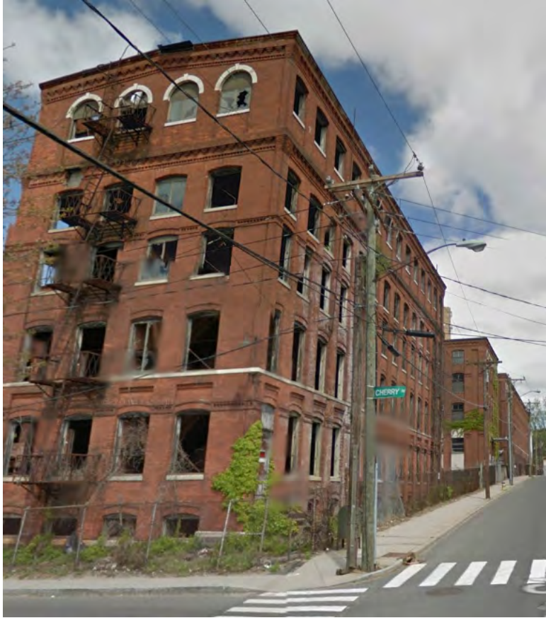
Figure 5. 177 Cherry Street (Buildings K and L, vacant) (Google Earth, 2015)
