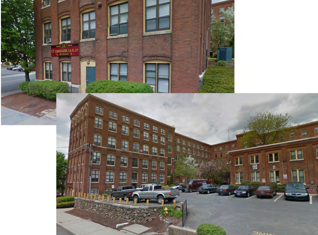
Figure 3. 13 Cherry Avenue (Buildings A, B, C, D, F, and M; Enterprise Apartments) (Google Earth, 2015)
