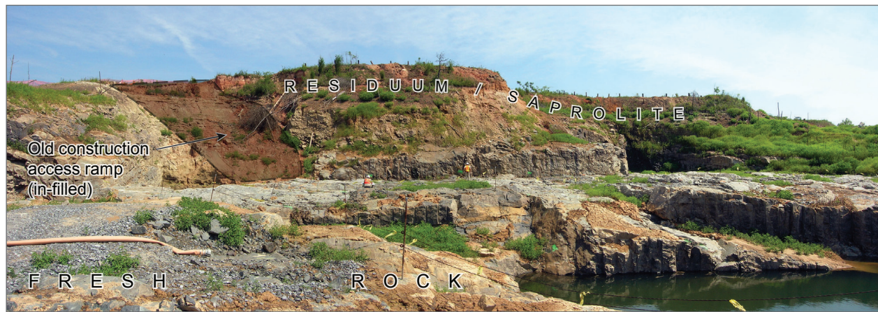
View north from center of former Cherokee nuclear site Unit 2
