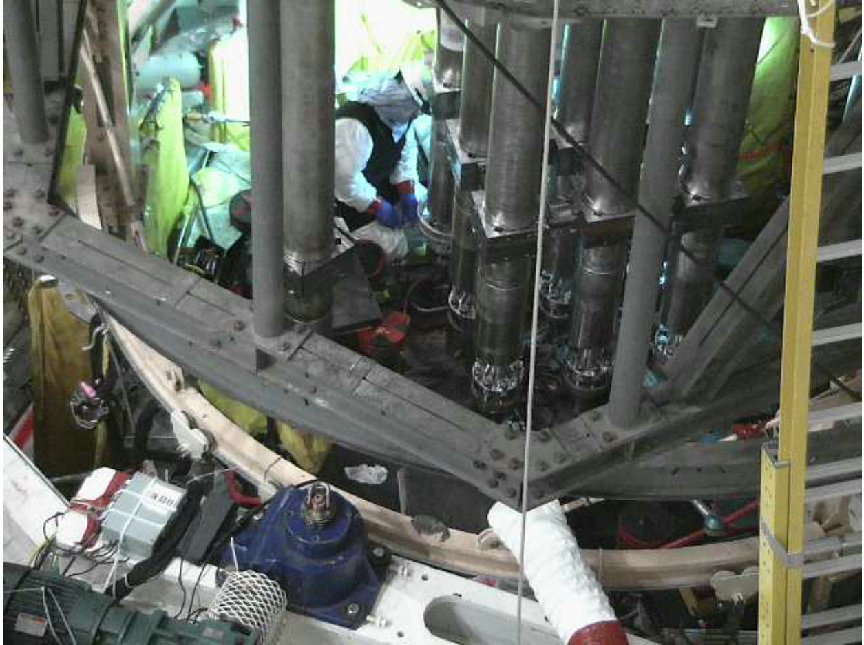
Worker at 11 o'clock wearing a shield vest with an apparent gap between the front vest and side back vest and appears to be seated.
