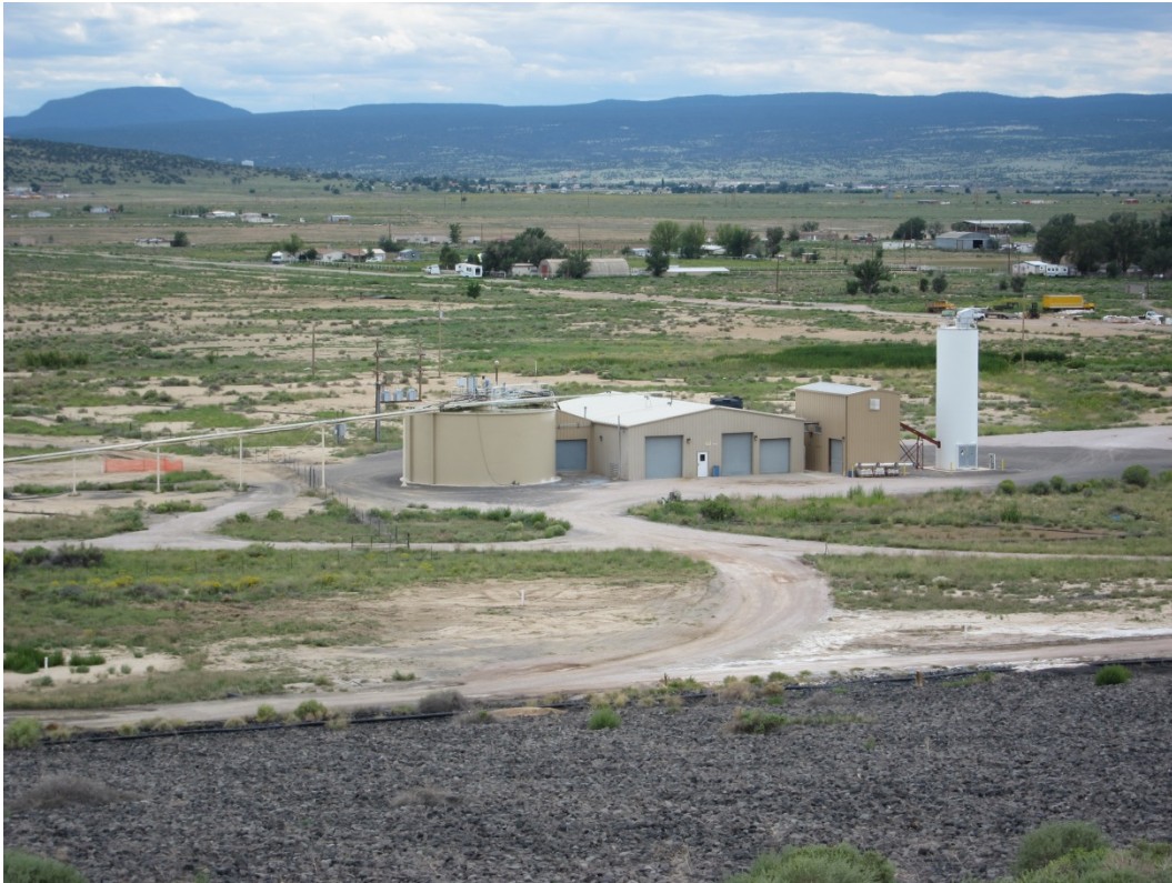
Figure 3: Water treatment facility in service with reverse osmosis equipment
