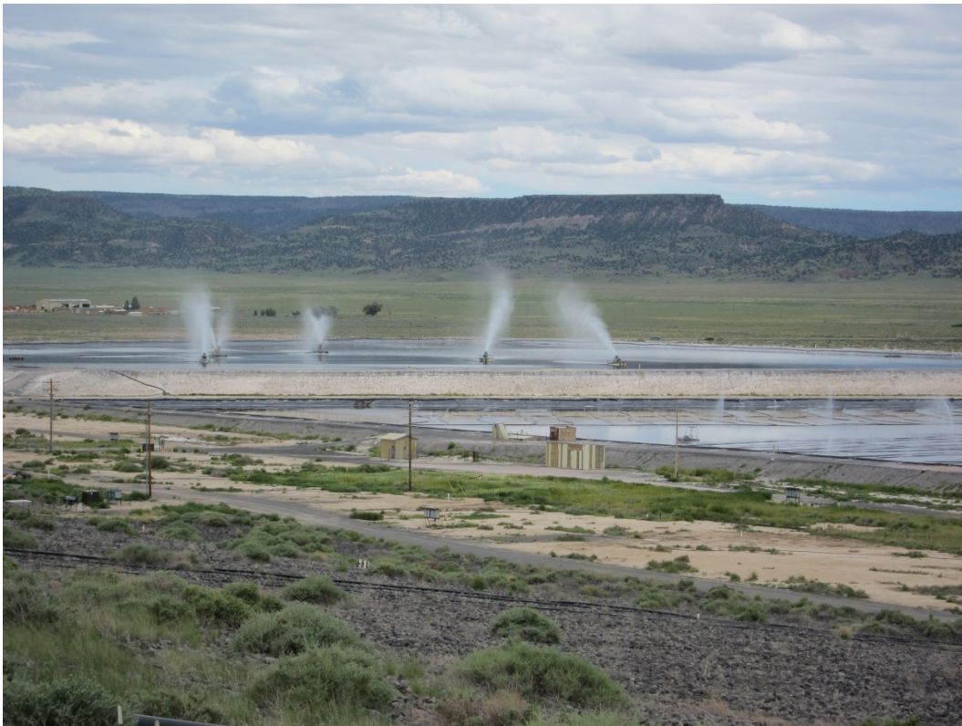
Figure 4: Evaporation pond sprayers in service
