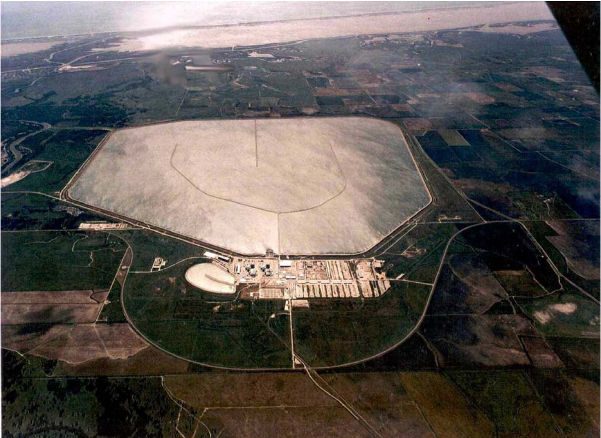
Figure 2.1-4 Oblique Aerial Photograph of STP Site
