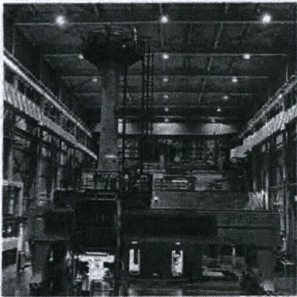
FIGURE 50 This fuel handling machine at the Hallam Nuclear Power Facility near Lincoln, Nebraska is used to exchange new and spent fuel elements in the sodium-graphite reactor located beneath the circular control rod mechanism housing (bottom center of photo). The mast is heavily shielded to protect plant personnel from the high degree of radiation given off by fuel elements withdrawn from the reactor for transfer to storage cells.
