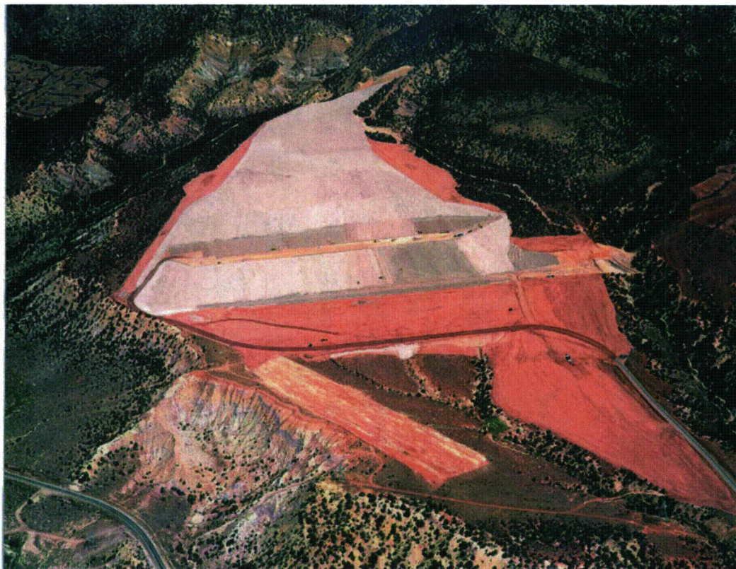
Photo 4. View north of Rifle disposal site during construction in 1994
