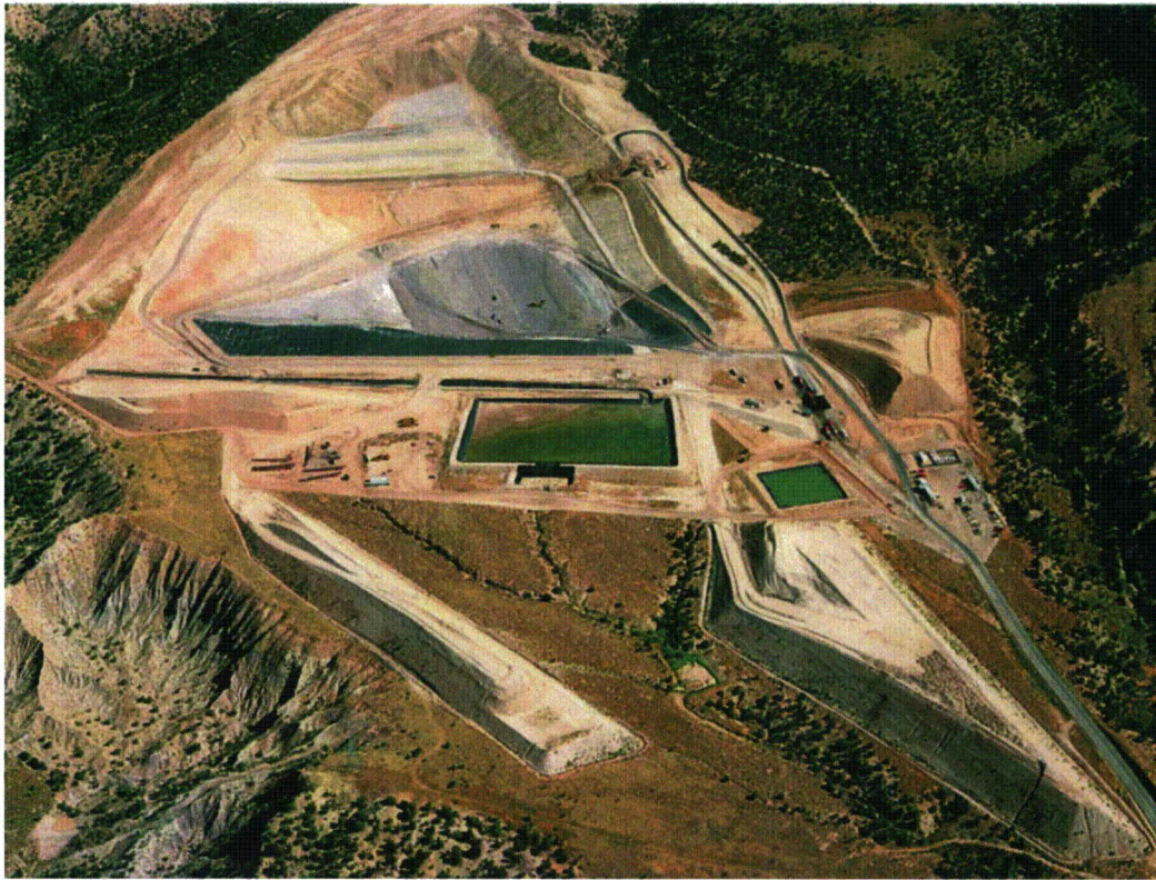
Photo 3. View north of Rifle disposal site during construction in 1992
