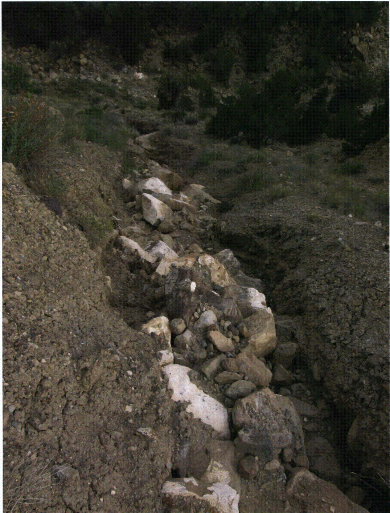
Photo 16. View downslope of the actively eroding gully within Unit 4 transmitting runoff from the Catchment Area (Unit 6) to the offsite natural drainage way
