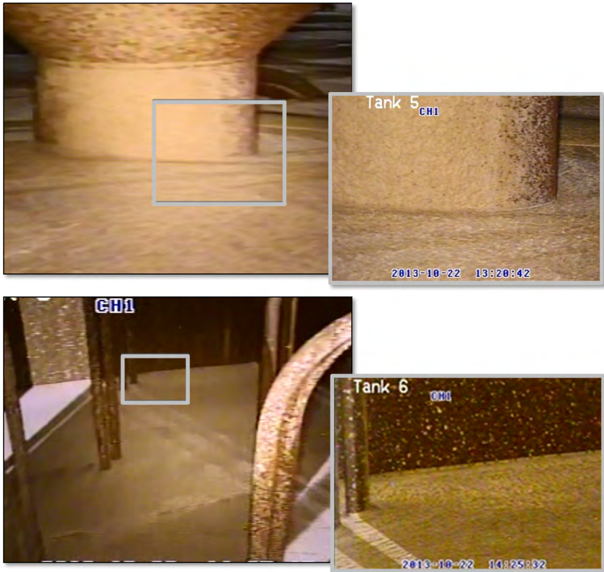
Figure 3.2-4: Grout Conditions on October 22, 2013, in Tanks 5 and 6 after Suspended Grout Operations
