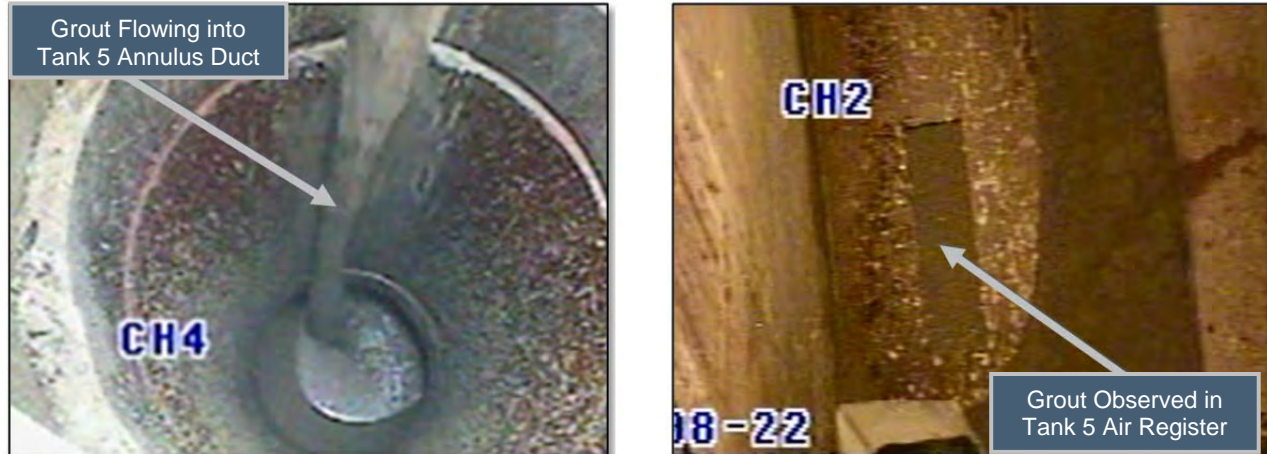
Figure 3.2-5: Grouting the Tank 5 Annulus Ventilation Duct (Lift 3)
