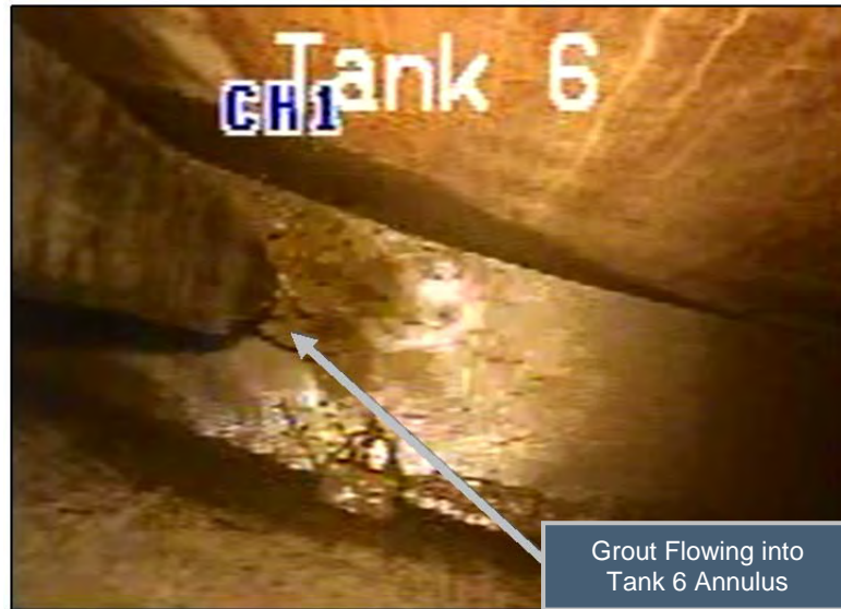
Figure 3.2-6: Annulus Bulk Fill Grout in Tank 6 during the Filling Process (Lift 5)
