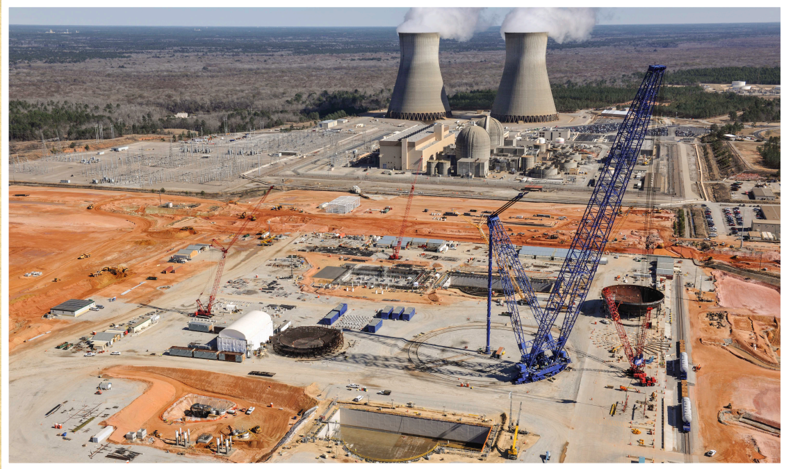
New Reactor Construction Site
