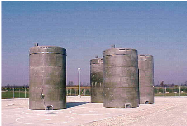
Spent Fuel Dry Storage Casks
