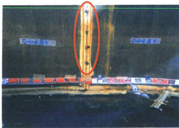
Sticking out of packing from a vertical flange part in the lowest side-plate layer (Photographed on September 19, 2013)
