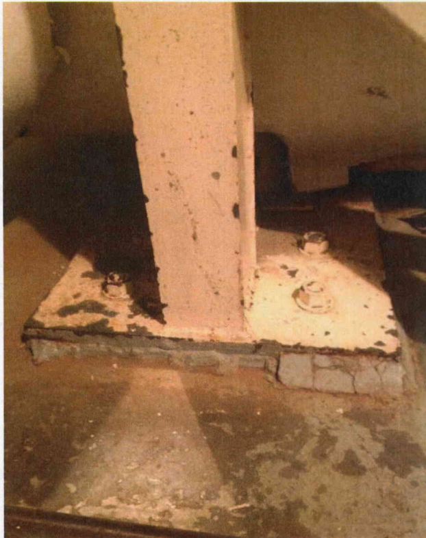
Photo 1 Damaged Grout
