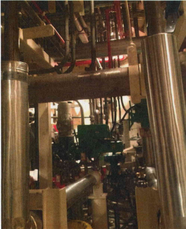
Photo 1 General View of Room 236
