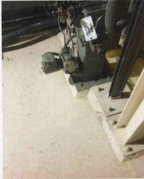
Photo 1 Damaged Grout
