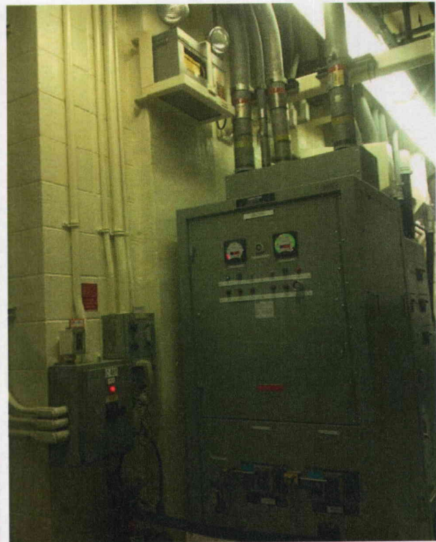
Photo 2 Masonry Wall Adjacent to Components
