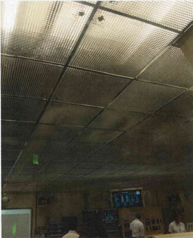
Photo 1 Ceiling Tiles and Lighting Fixtures Anchored
