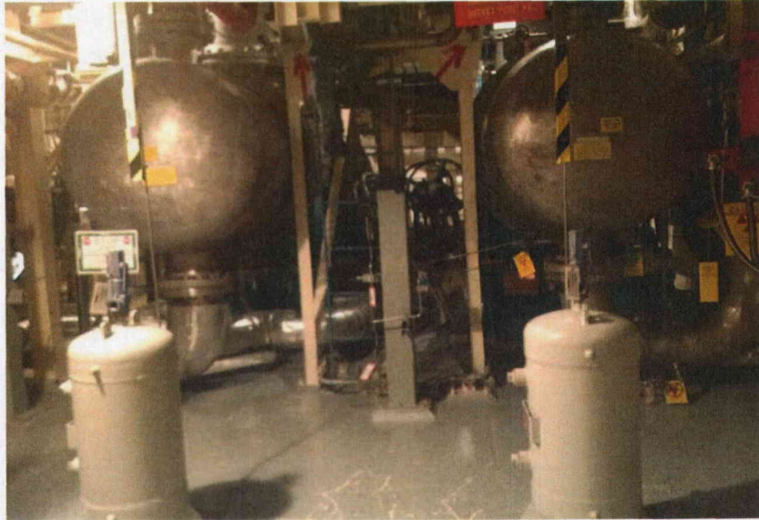
Photo 1 General View of Room 113
