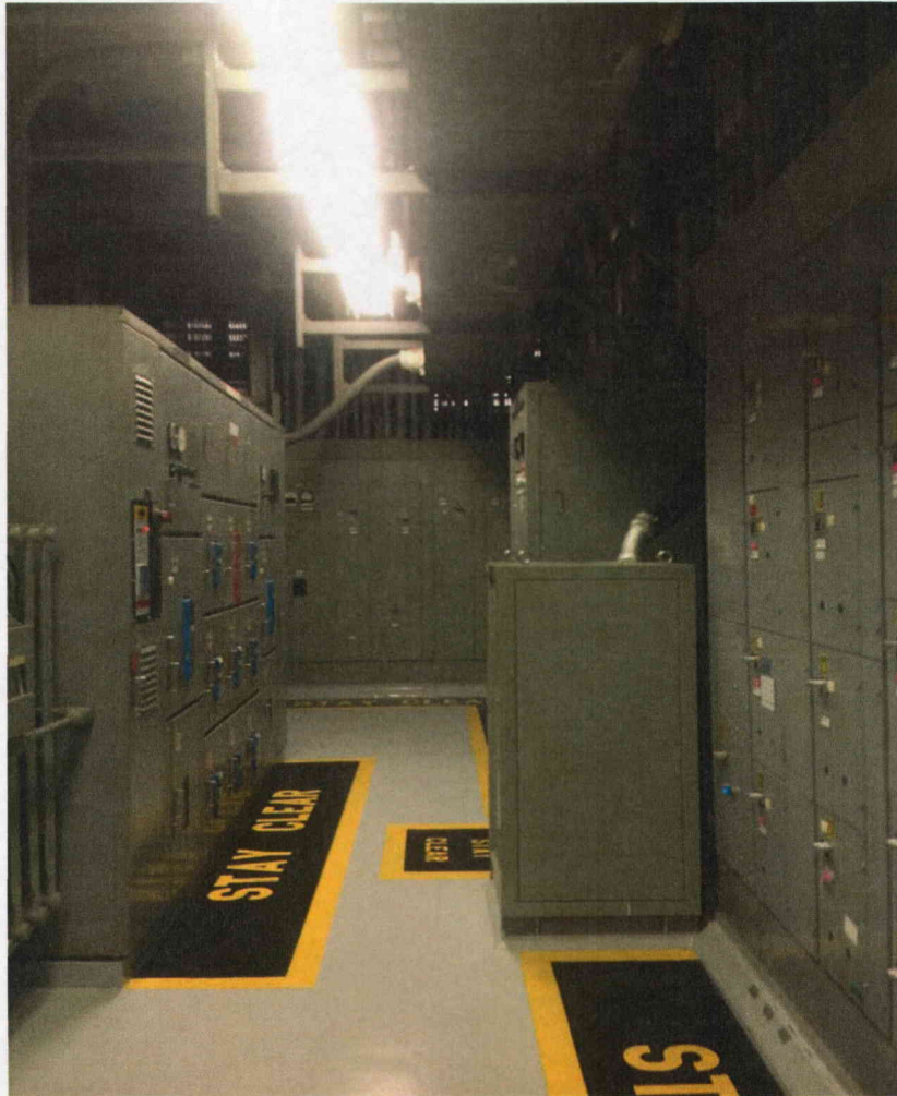
General View of Room 429
