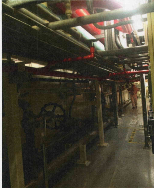
General View of Room 304
