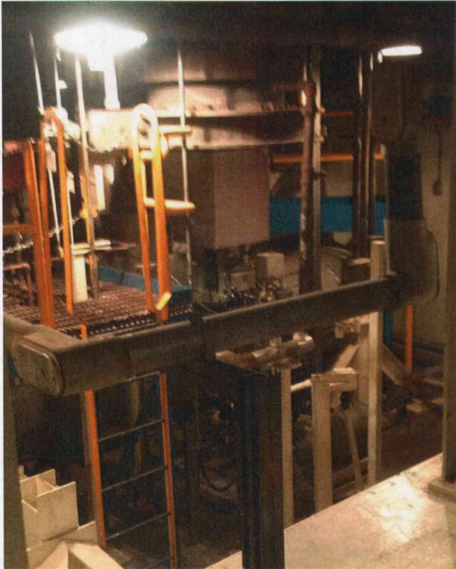
Photo 1 General View of Room 602
