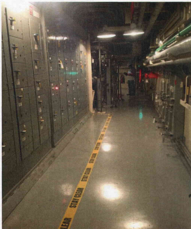
Photo 1 General View of Room 209
