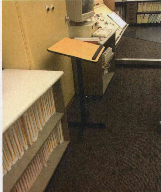
Photo 2 Small Podium Not Anchored
