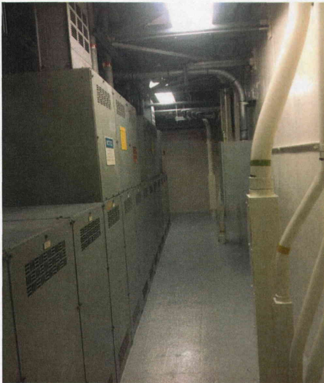
Photo 1 General View of Room 323
