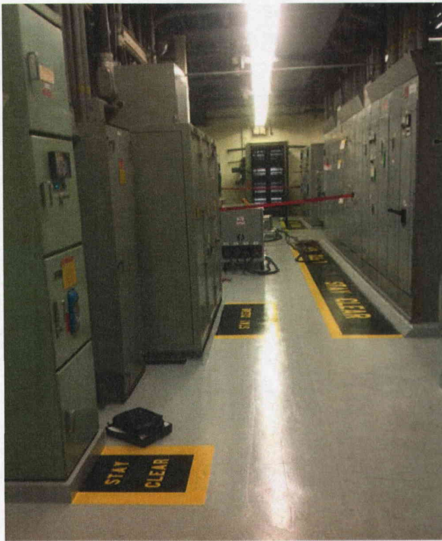
Photo 1 General View of Room 428
