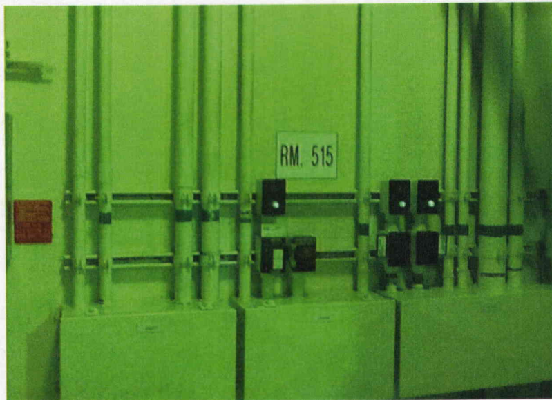
General View of Room 515
