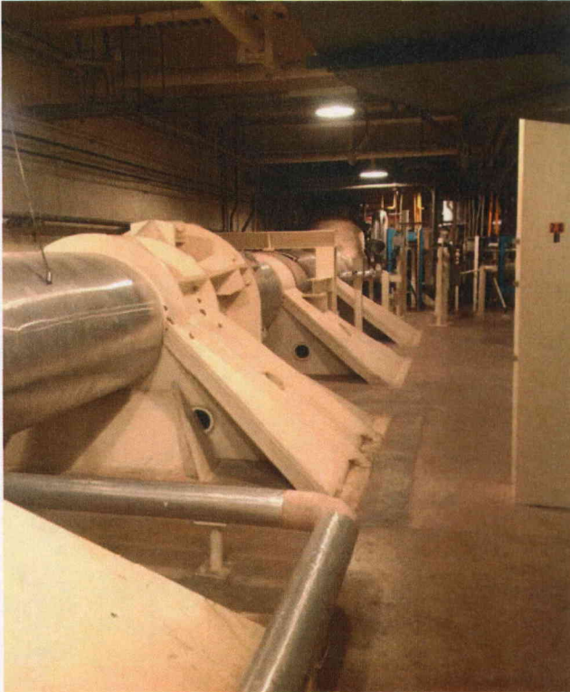
Photo 1 General View of Room 601
