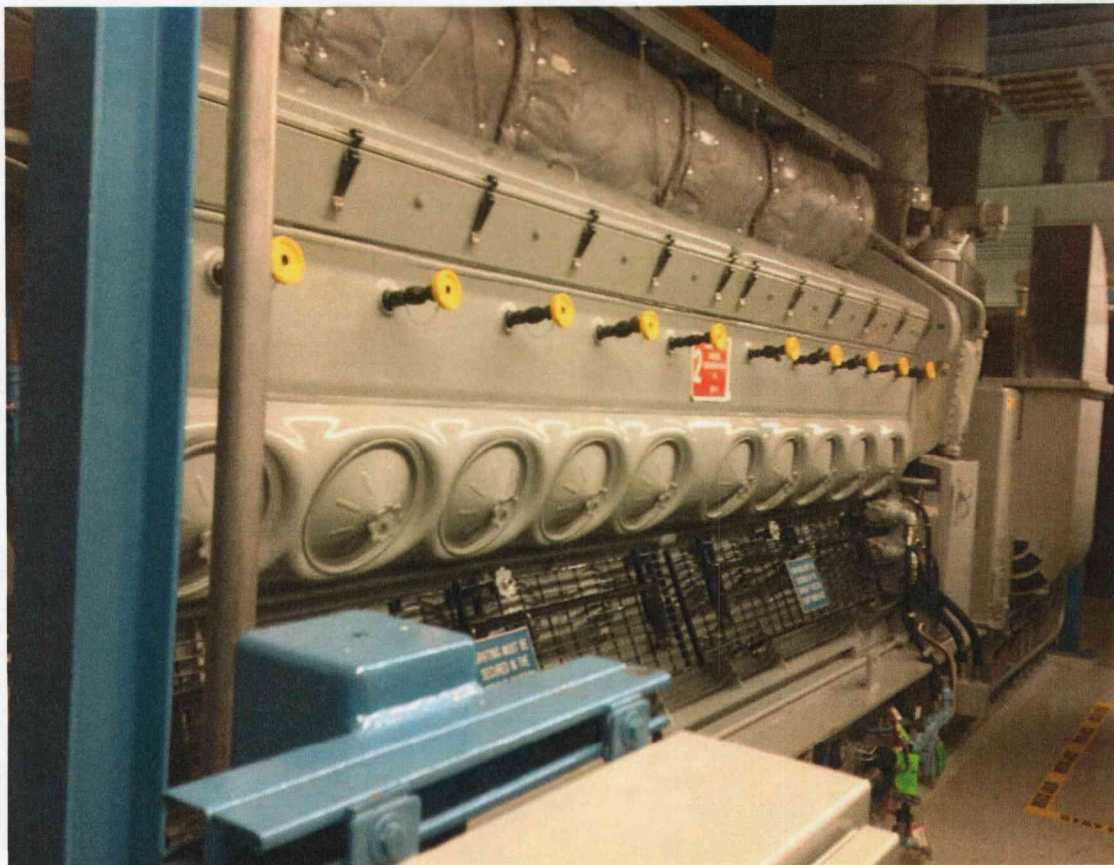
Photo 1 General View of Room 319
