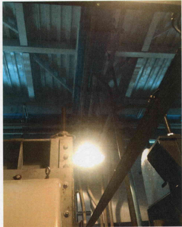
Photo 2 Rod Hung Pipes
