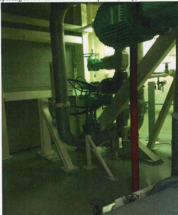
Photo 1 General View of Room 303
