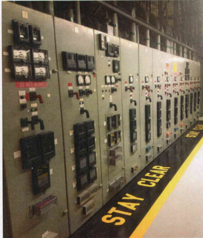
General View of Room 325
