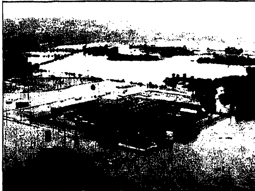
Fort Calhoun Aerial Picture of Flooding
