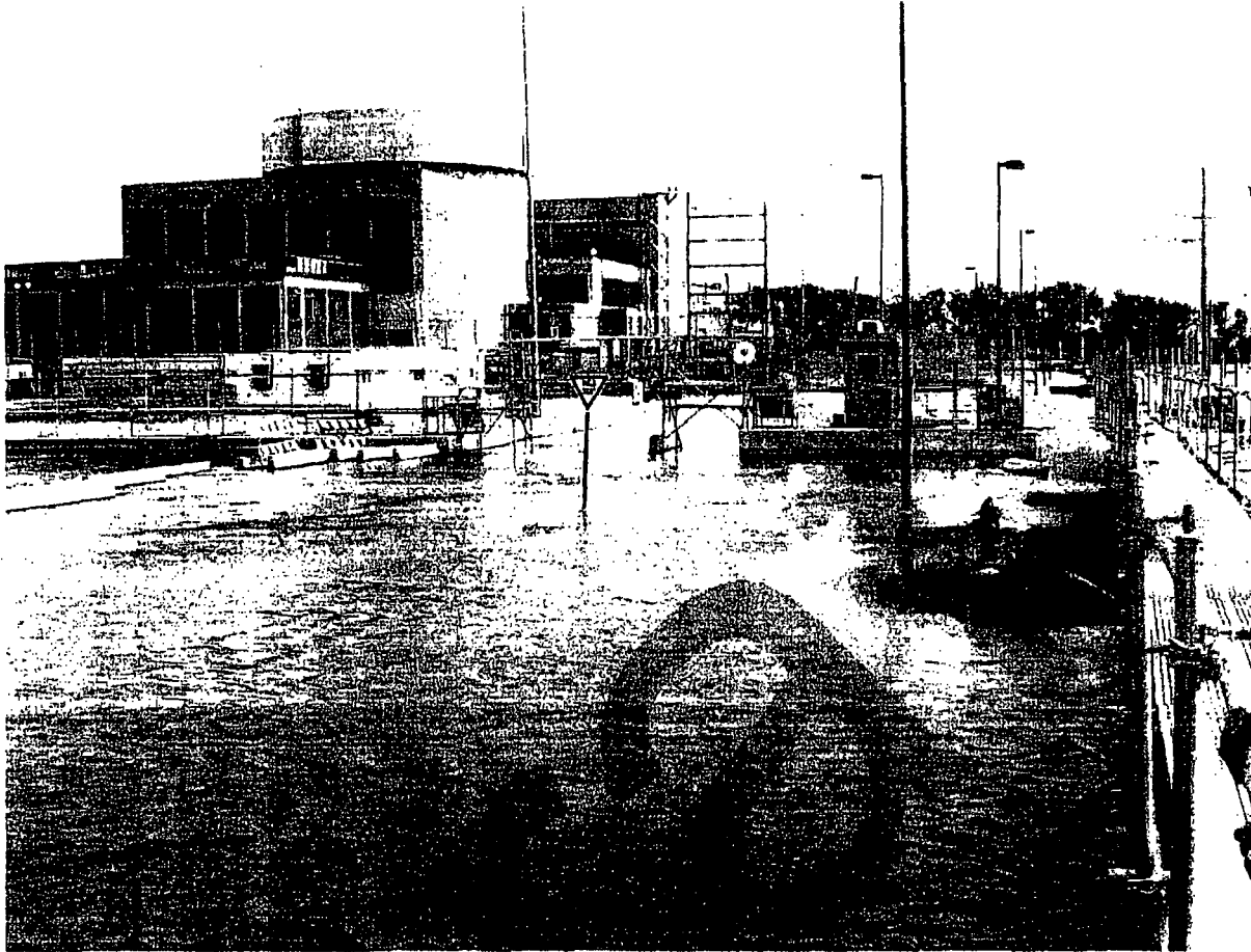
Photo 2 – Floodwater at FCS, Looking East toward the Containment
