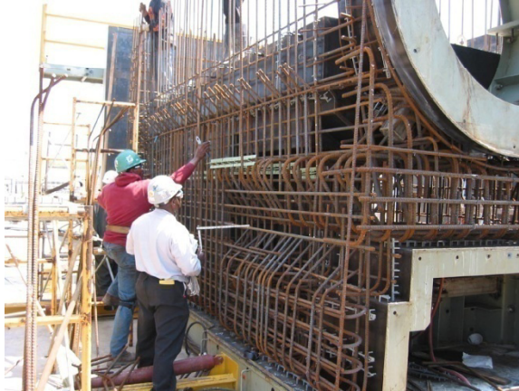
Horizontal Storage Module under construction
