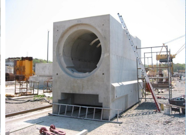
Horizontal Storage Module under construction
