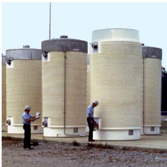
Figure 2-1. Dry Storage of Spent Fuel (Source: NRC 2012a)
