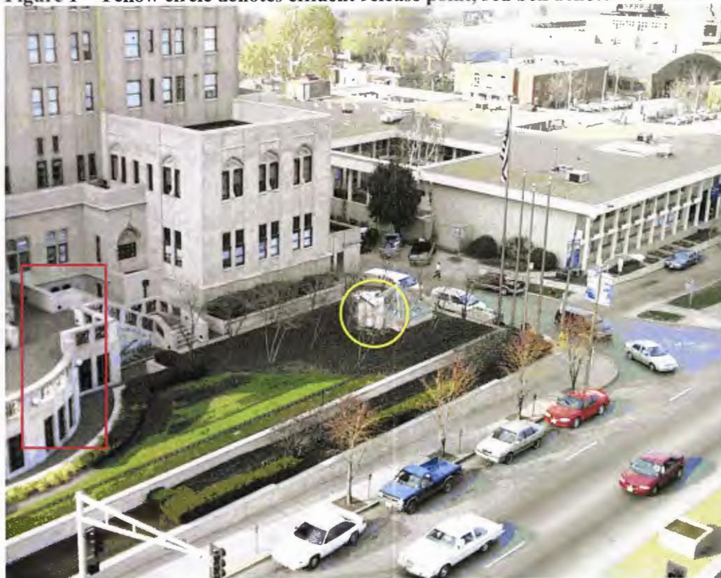
Figure 1 – Yellow circle denotes effluent release point, red box denotes deck area
