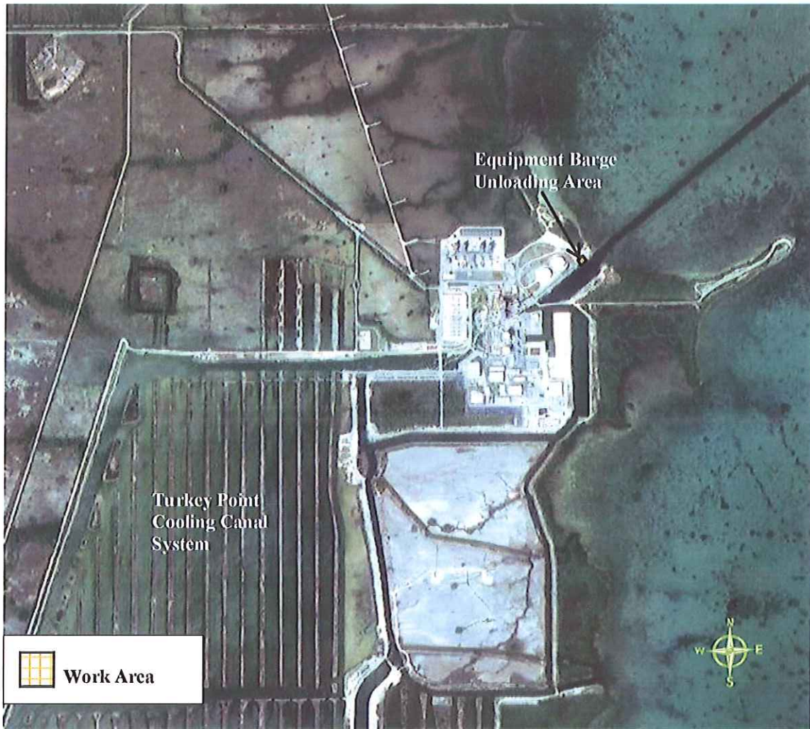
Figure 9 – 1: Turkey Point Units 6 & 7 Equipment Barge Unloading Area
