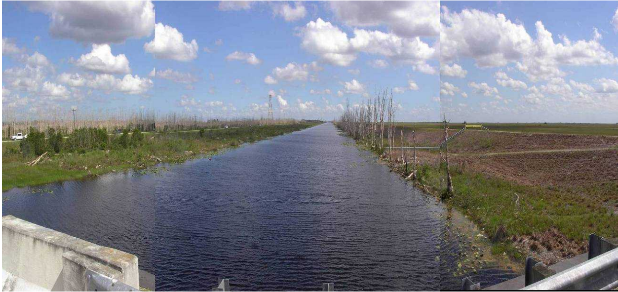
Photo 4. Levee Along Krome Avenue (June 2005)
