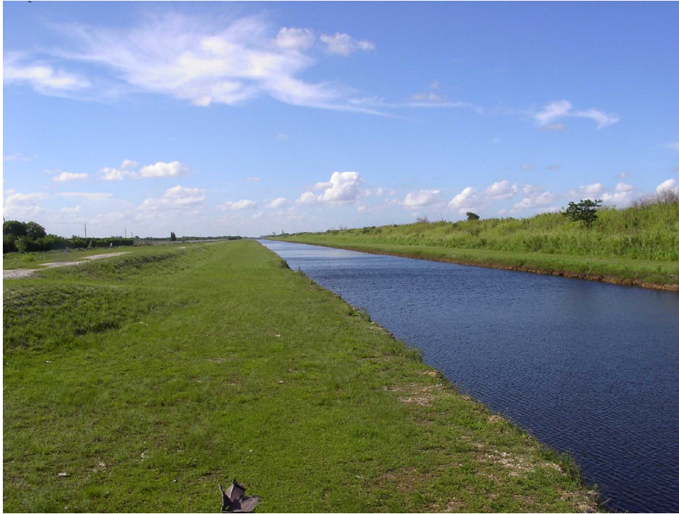
Photo 5. Canal and levee with agricultural lands to the west. This photo is near the Howard Drive crossing of the levee, into the largest agricultural area outside of the levee system. June 2005.
