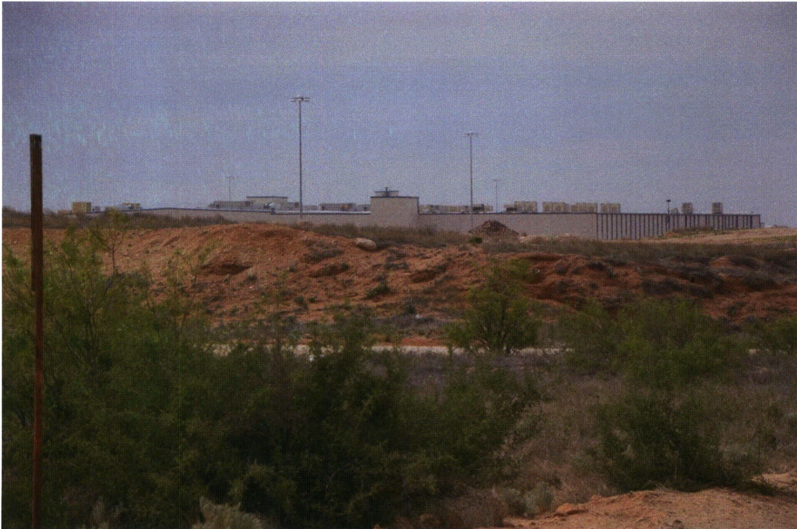
Figure 3.9-1D URENCO USA Facility as Seen From the Northern Property Boundary Looking South. (Photograph Taken 26 April 2012)
