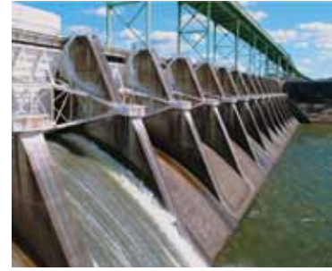
Water spills over the Fort Loudon Dam in Loudon County, Tennessee.
