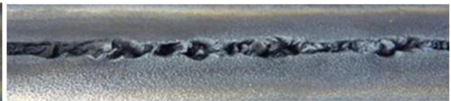
Unshielded Backside Weld
