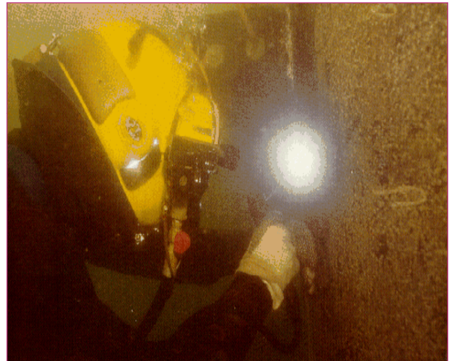
Underwater welding with SMAW
