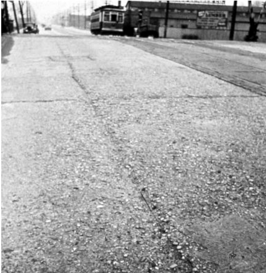
North Lanes Constructed With Non Air-Entrained Portland Cement
