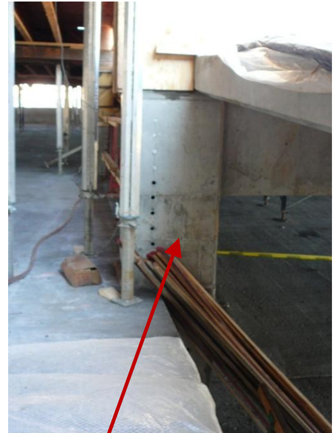
Crack in Column
